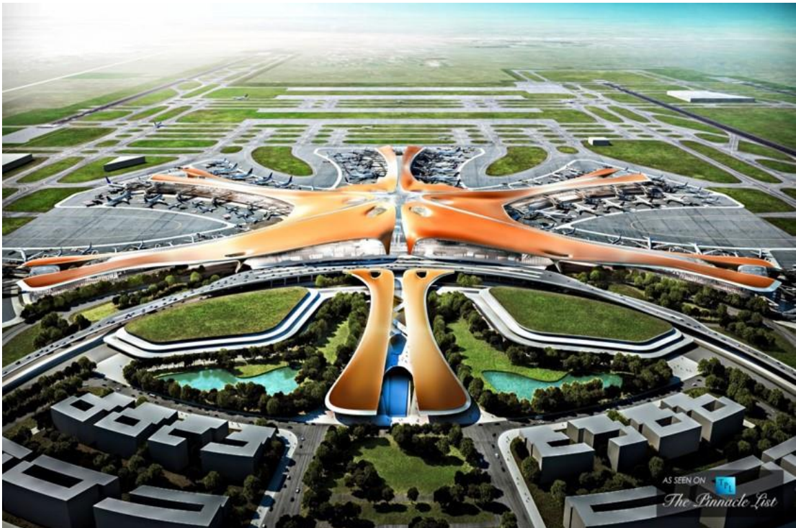
Figure 11. Exterior of Beijing Daxing Airport ( www.zaha-hadid.com )
