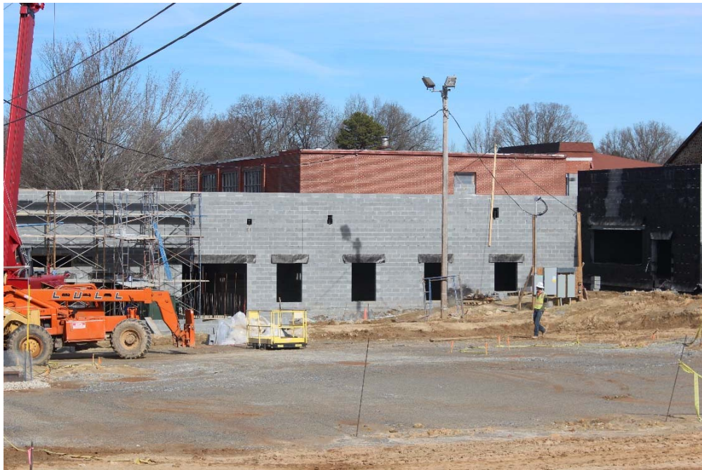
Figure 26. New Construction Continues at the Academy.
