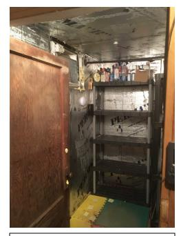
A room in the basement was converted into a walk-in cool room using a CoolBot controller, rigid insulation, and a window A/C unit. While the Carrows consider the equipment on their operations to be maximally efficient in their energy use, they are interested in solar photovoltaics for generating electricity, specifically for running a fan in the greenhouse that currently has no power, and for their water pumping needs.
