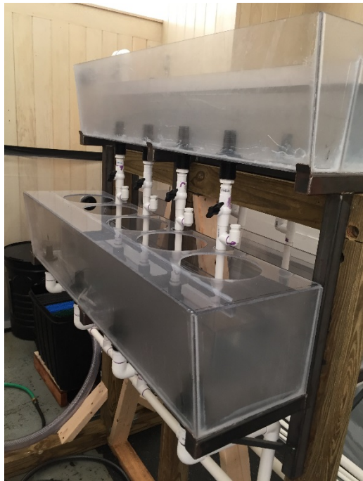
Figure 5. Modified vertical flow greywater processing unit.
