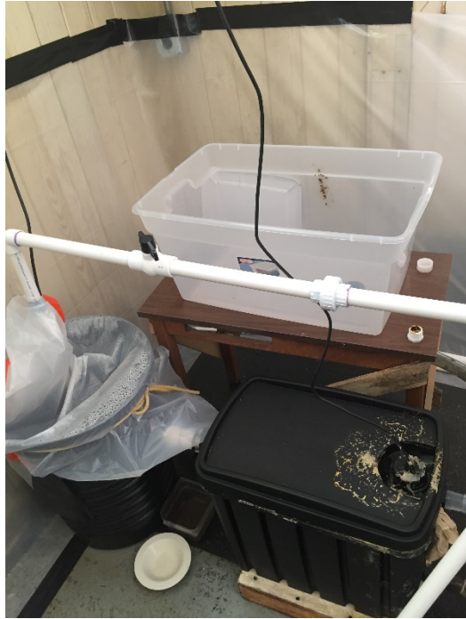
Figure 4. Sump tank and biofilter units.
