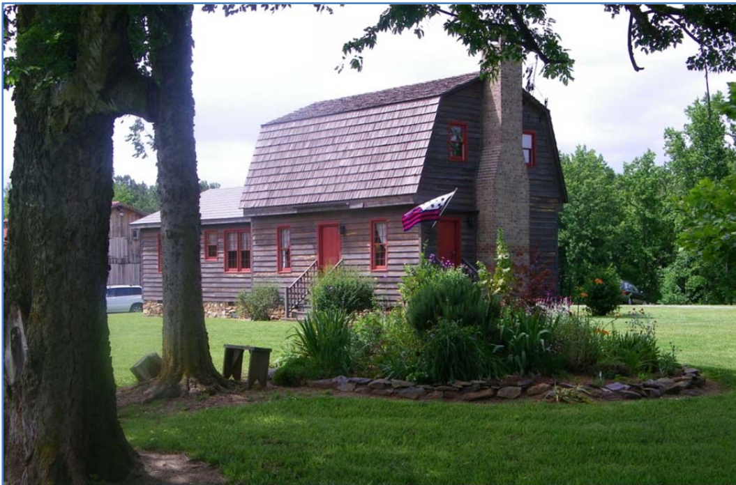
The reconstructed 1755 John Brooks house with the handiwork of master gardener Dawn Gilmore in the foreground. The gambrel roof was unusual in this region, as were the glass windows.
