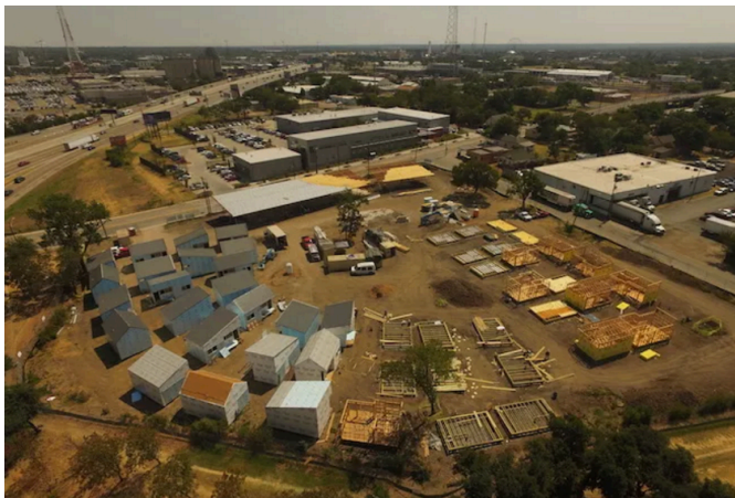
Figure 11: The Cottages in construction in Dallas.
