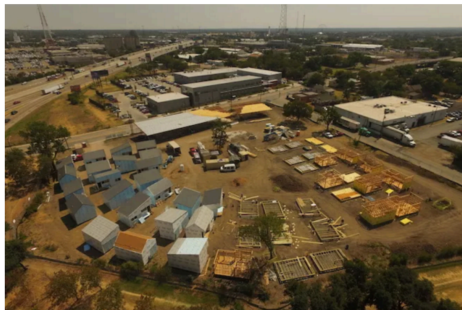
Figure 11: The Cottages in construction in Dallas (Carlyle, 2014).
