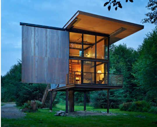
Figure 7: The Cabin on Stilts; a 350 square foot static tiny home.
