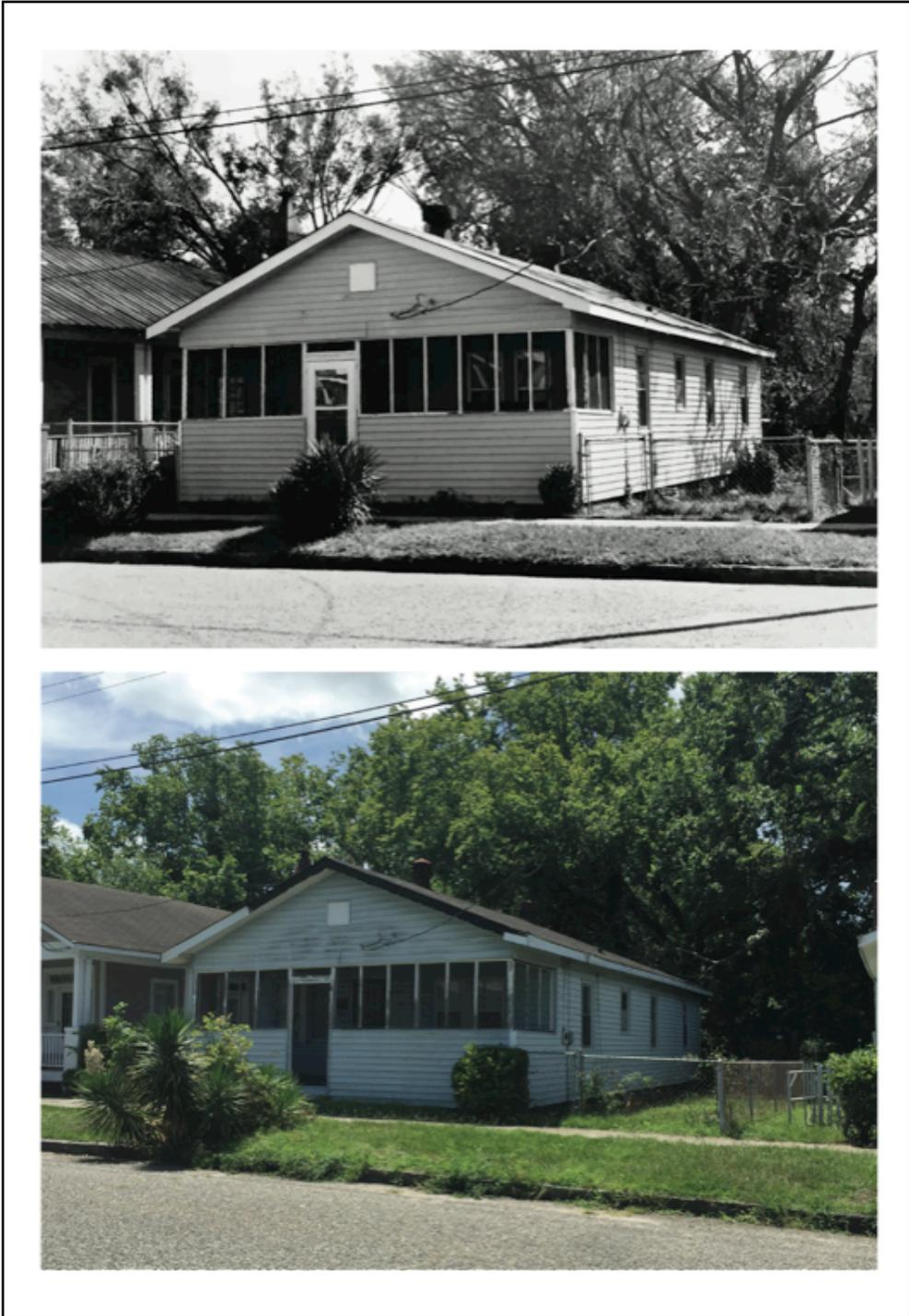
**Figure 26. Northside, Site #28, Coded as Deteriorated.** Top image, archival photograph. Bottom image, photograph taken Summer 2015. Field notes: Noticeable exterior wear and tear. Missing part of gable. Needs cleaning.
