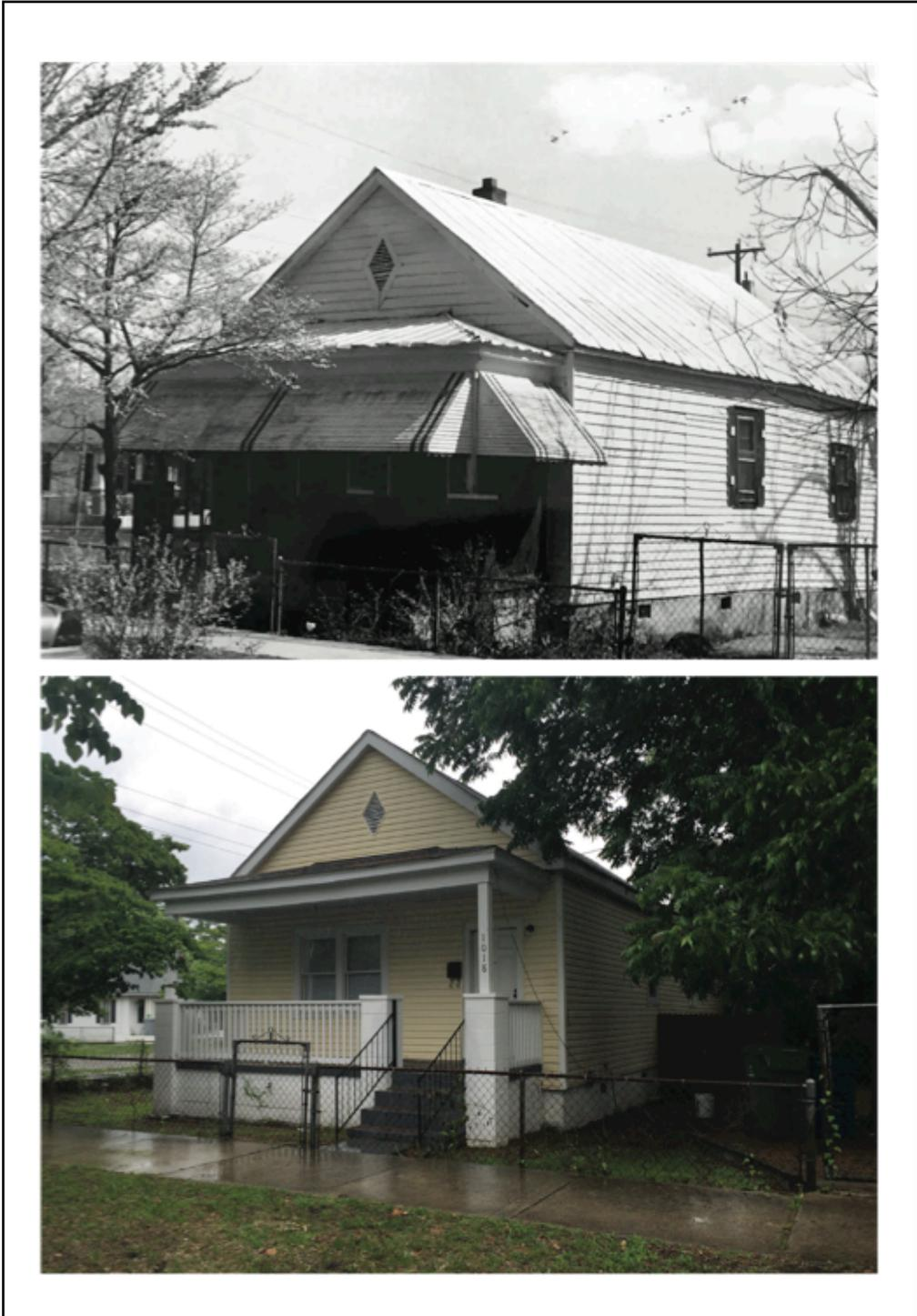
**Figure 28. Northside, Site #4, Coded as Rehabilitated.** Top image, archival photograph. Bottom image, photograph taken Summer 2015. Field notes: awning off, replacement windows, yellow vinyl siding and a new shingle roof.
