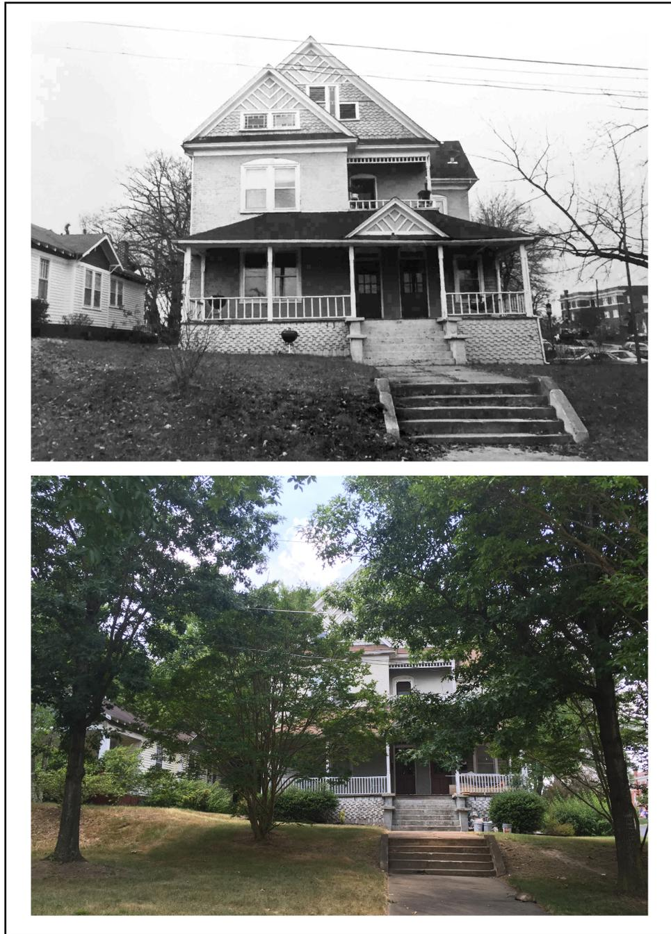
**Figure 10. College Hill, Site #15, Coded as Deteriorated.** Top image, archival photograph. Bottom image, photograph taken Summer 2015. Field notes: Jackson street. Replacement windows. Structure needs paint. Balustrade at top falling off. Shingles missing. Deteriorating. See Appendix F for supplemental photograph to support field notes.
