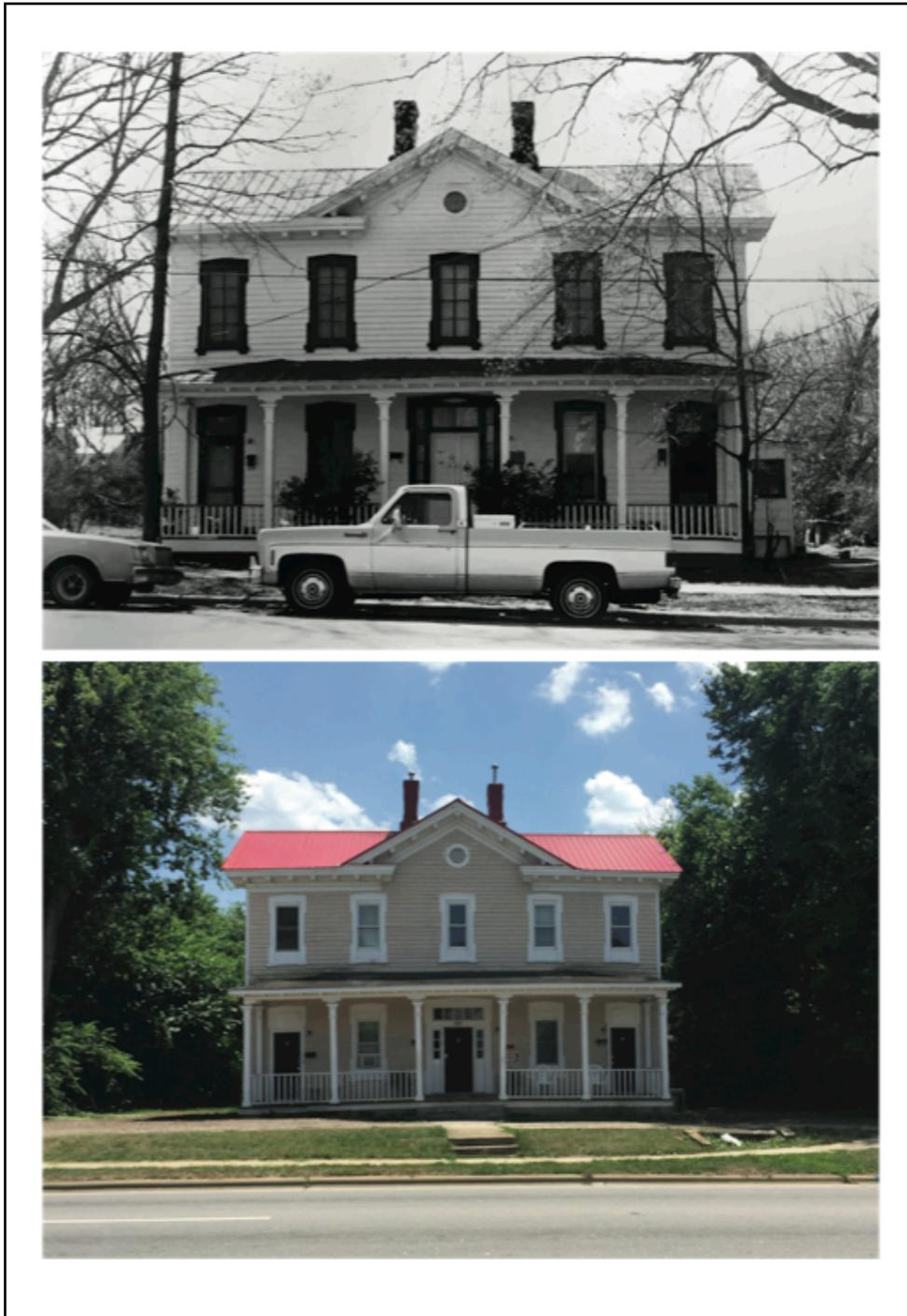
**Figure 23. South Park, Site #13, Coded as Rehabilitated.** Top image, archival photograph. Bottom image, photograph taken Summer 2015. Field notes: Replacement windows. Otherwise rehabbed with fresh paint and new roof.
