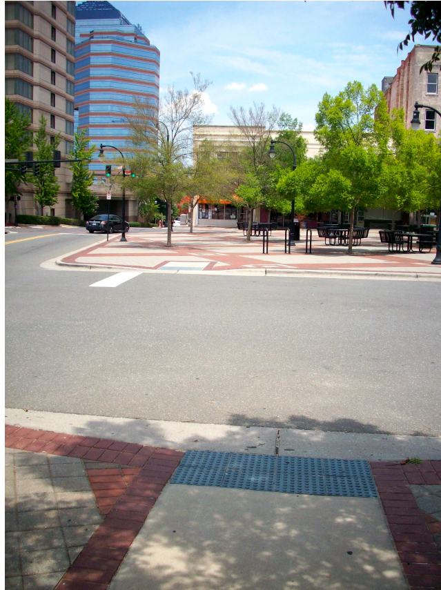
Figure 5. Point 9 marked on Figure 3. This figure shows the lack of crosswalk at CCB Plaza.
