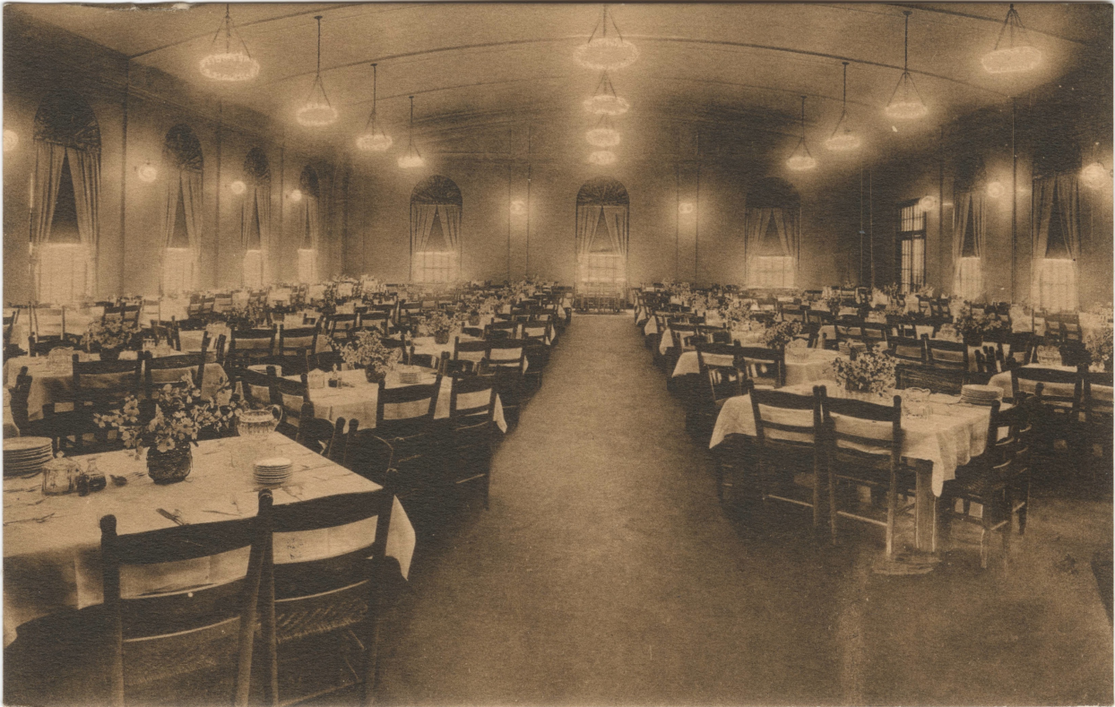
Figure 6. “Beautiful” and “attractive” lighting in the dining hall as described by Edith Bollinger in 1922.
