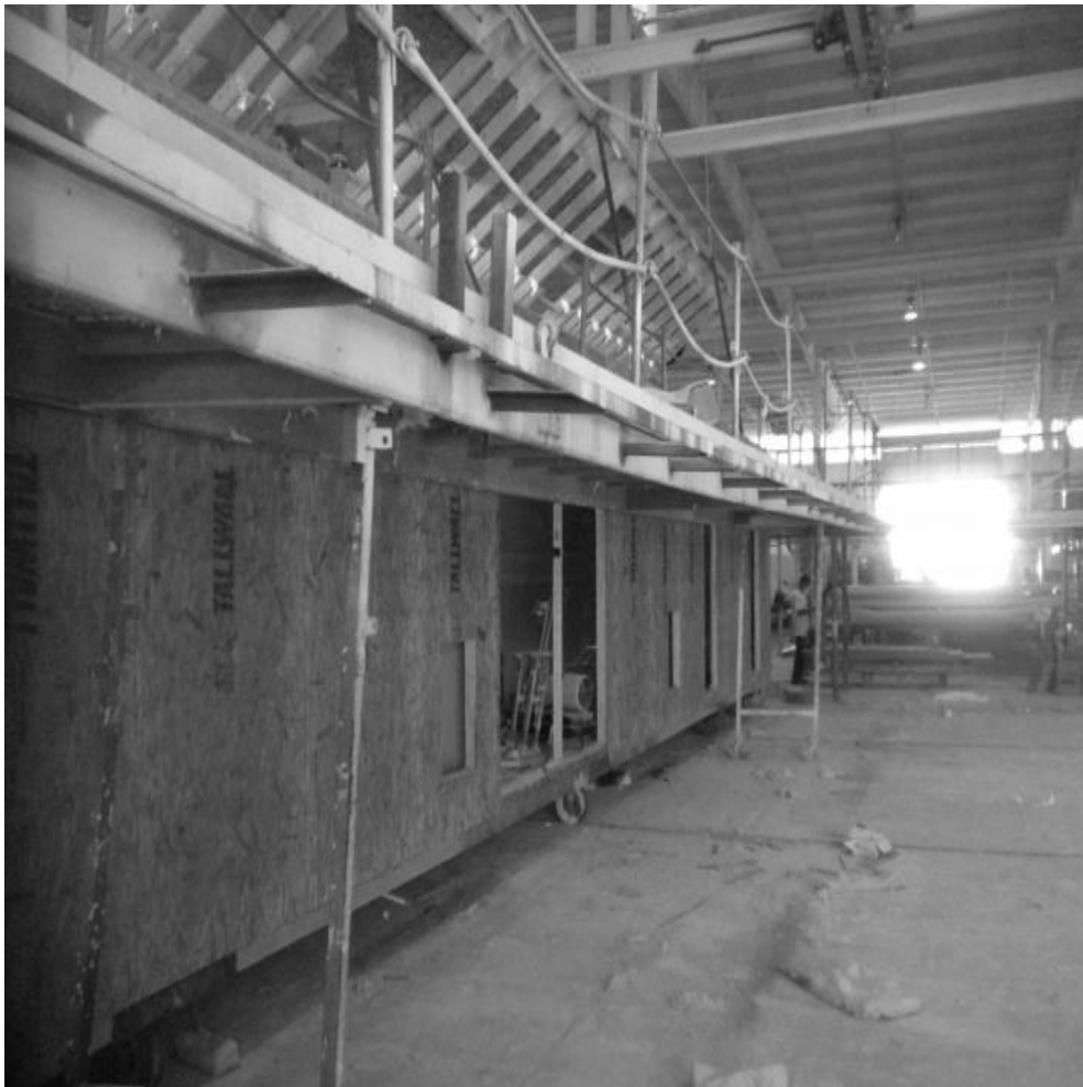
Figure 7. Factory floor of Carolina Building Solutions, a North Carolina-based manufacturer of modular buildings (photo by author).
