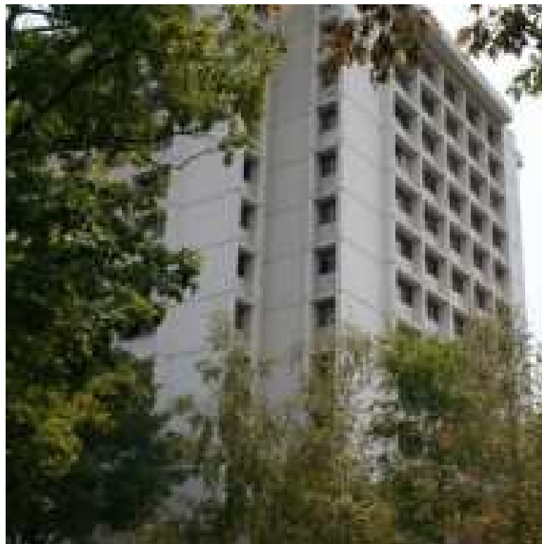
Figure 23. Holshouser Hall at UNCC, one of the cast-in-place concrete buildings from 1972 currently being fully renovated (UNCC, 2014. Reprinted with permission).
