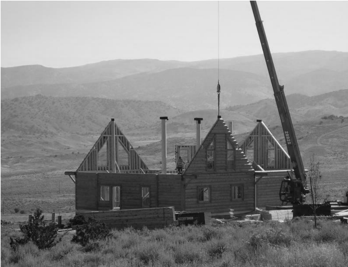
Figure 5. A panelized log-home kit that comes to the job site as panels and labeled components ready for assembly (Grizzly Log Builders, 2014. Reprinted with permission).
