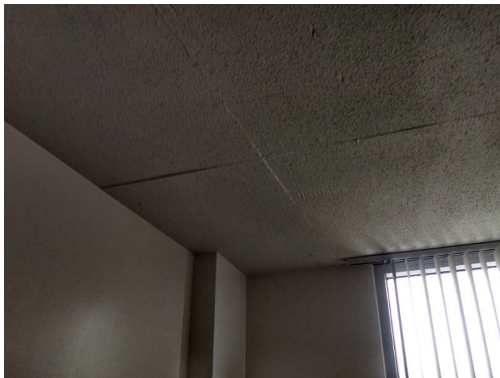
Textured ceiling inside of a Summit dorm room. Notice the patterns left by the formwork that the paint attempts to cover.
