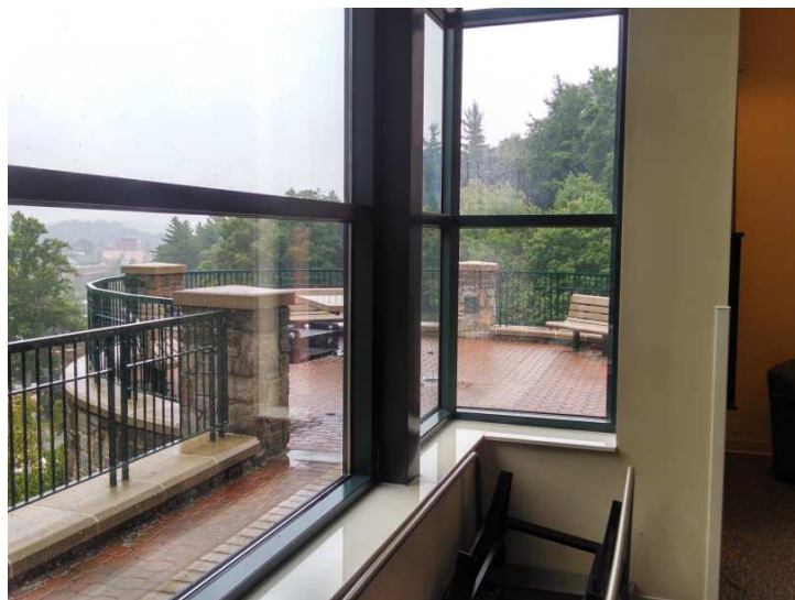
Traco window details with view of exterior courtyard constructed at Mountaineer.
