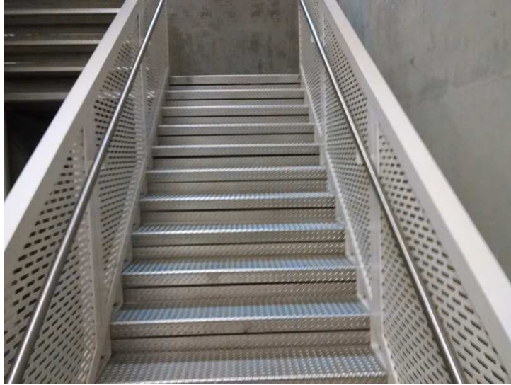
Another view of the Summit stairwell.
