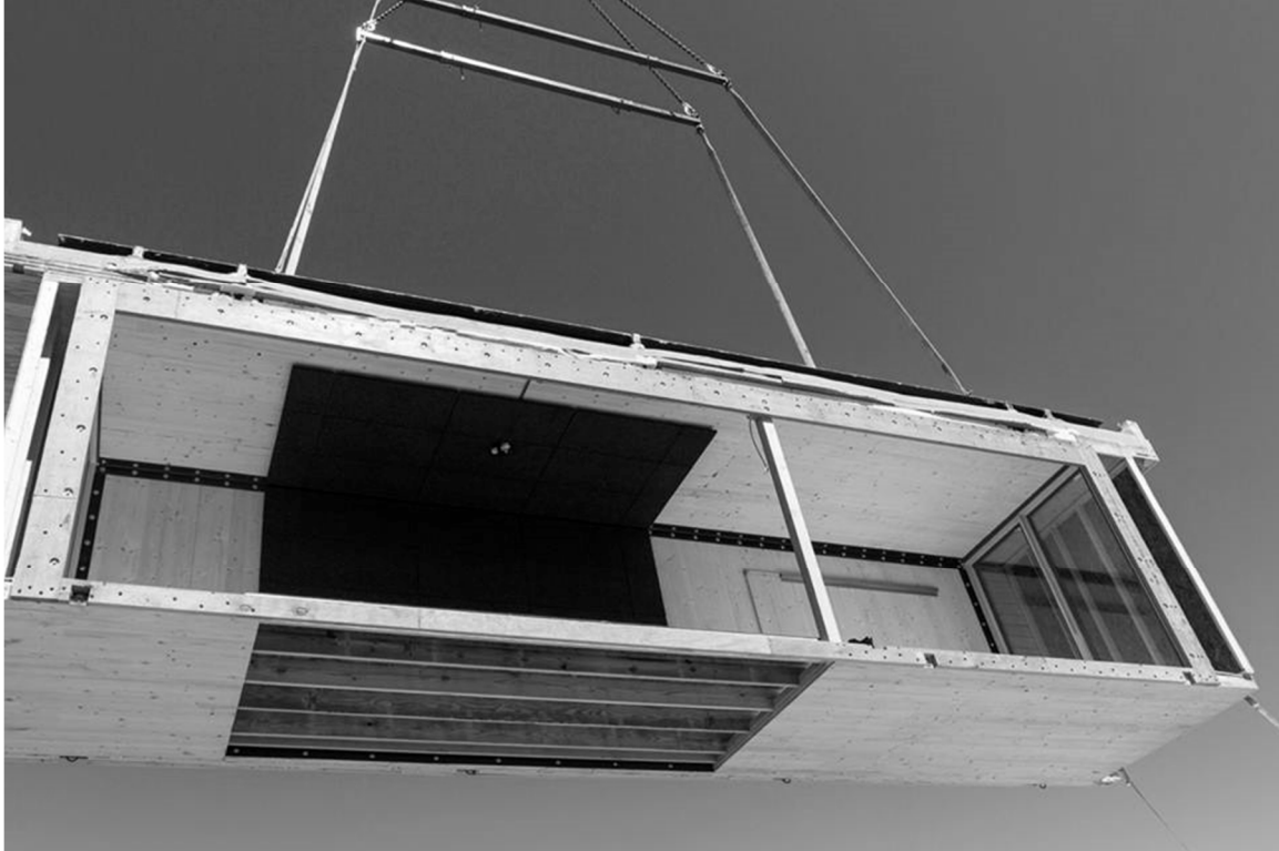
Figure 2. A building module constructed of CLT is removed from adjoining modules (photo courtesy of Dudley Carter).
