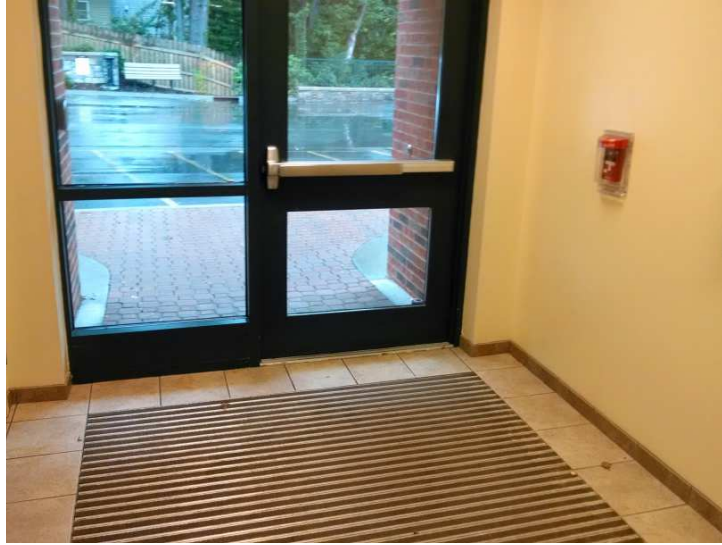
Entrance to Mountaineer hall with walk off grates to prevent tracking in dirt and moisture.
