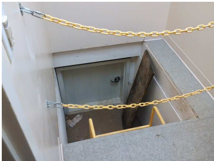
Crawl space access at Mountaineer.
