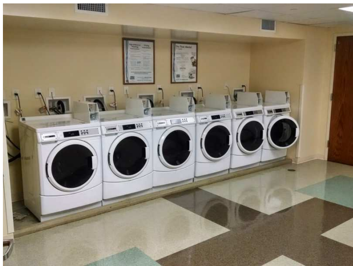
Laundry facility at Mountaineer that sends an alert to residents when their laundry has finished its cycle.
