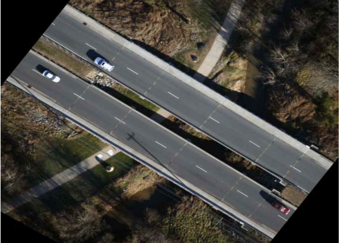
Figure 5.4 Mallard Creek bridge joint width quantification using aerial imagery
