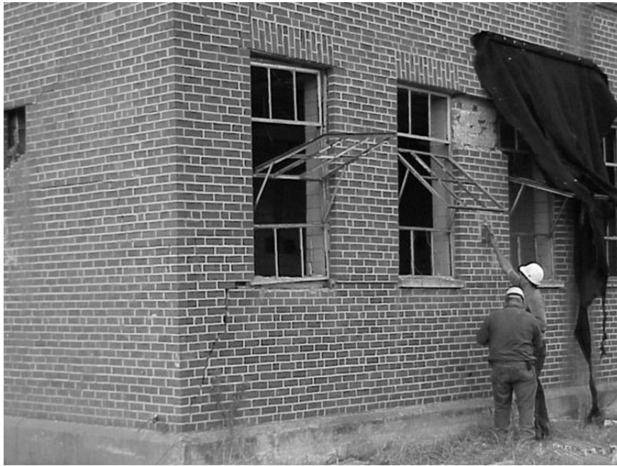
FIGURE 2.18: Post-test exterior view of intersection of Wall #3 and Wall #2. Note the area of spall on Wall #3 at upper right. The remaining geotextile fabric used to catch ejecta is visible at right.
