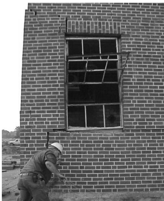
FIGURE 2.17: Post-test exterior view of Wall #3 where it intersects Wall #2.
