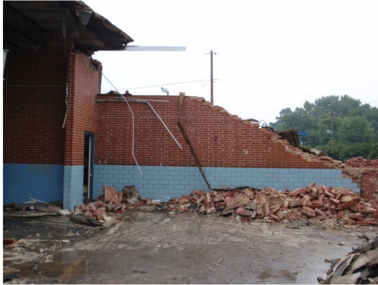
Figure 3-2: Demolition of the brick masonry walls at Idlewild Elementary School.
