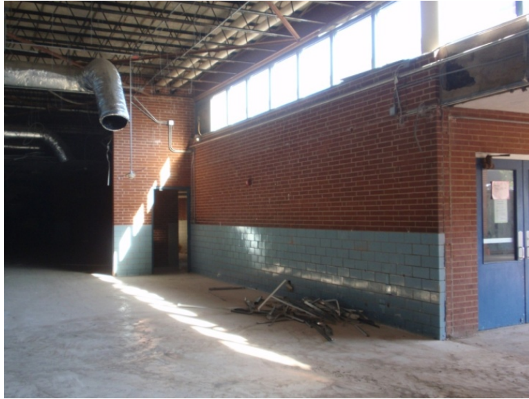
Figure 3-1: Cafeteria at Idlewild Elementary School prior to demolition.
