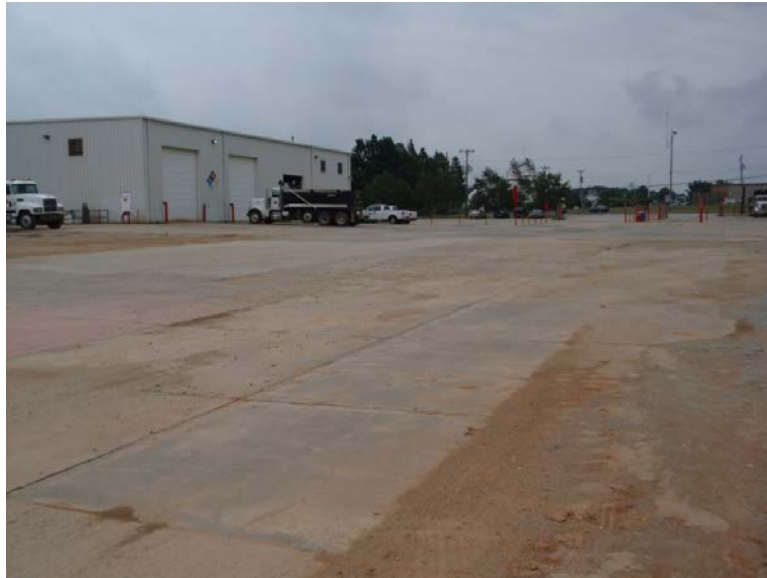
Figure 7-4: Overview of the proposed test pavement site.
