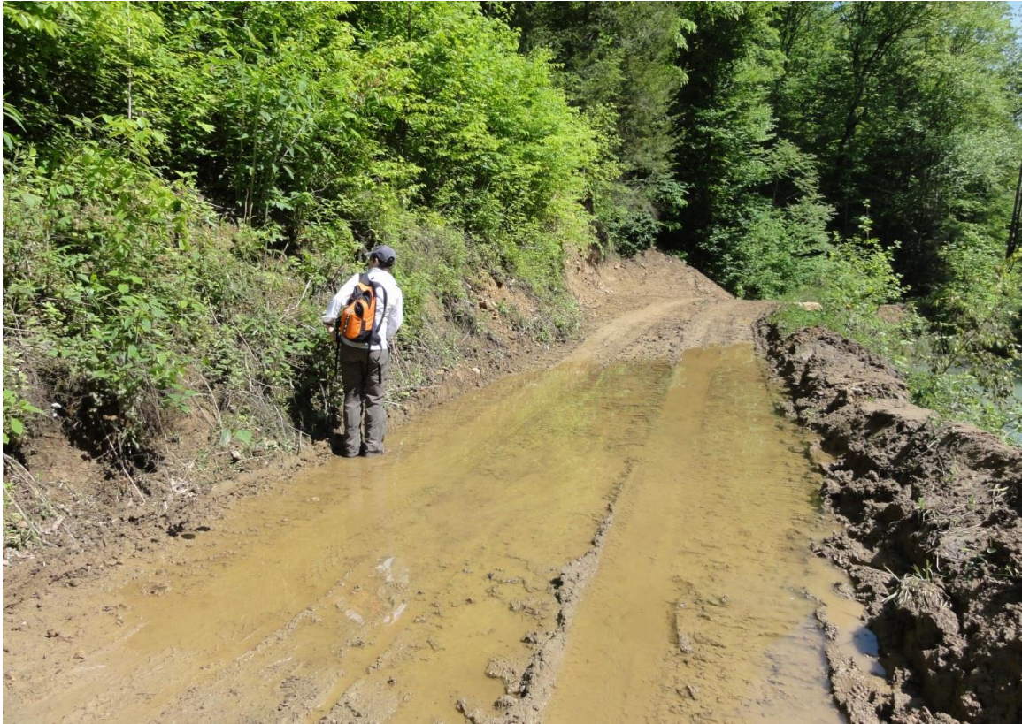
Figure 3.8. Site Visit Photo – Road at Base of Valley Fills
