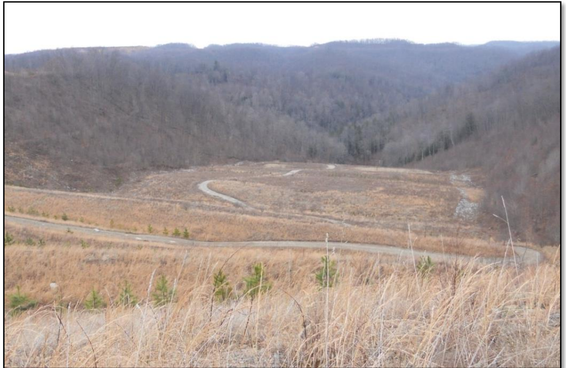
Figure 3.7. Site Visit Photo –Valley Fill 1
