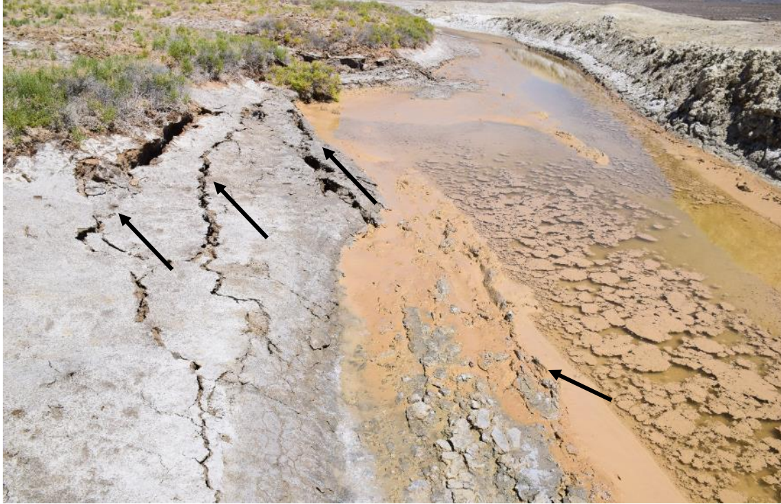
Figure S17. Lateral spread along banks of Salt Wells Valley. Active creek bank free-face failure due to seismic shaking from M 7.1 event. Lat. 35.651326°, Lon. -117.485338°. Photo 0408 credit J. Patton, CGS.
