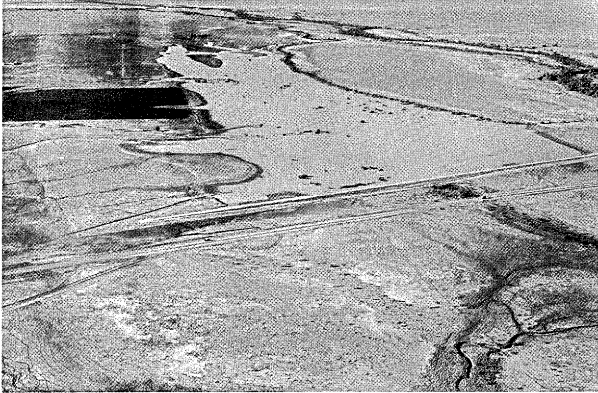
Plate VI: The Richmond Shallow Water Research Project dam near O'Connell Creek with adjacent cultivation irrigated from it.
