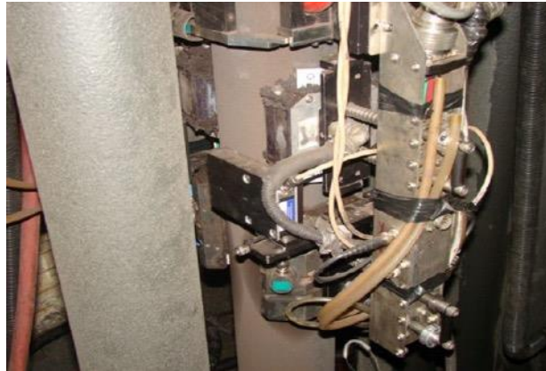
Figure 2-25 H-Scan® of Reformer Tubes [16]
