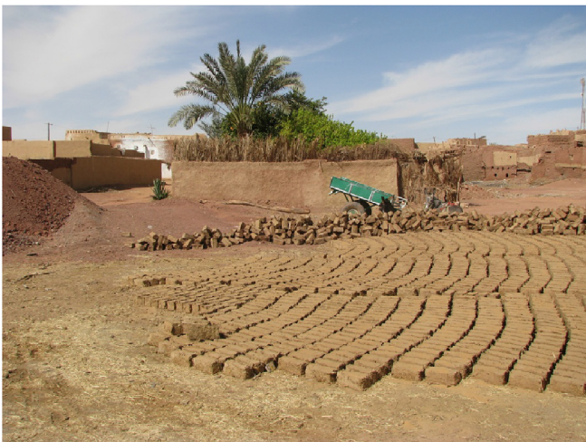
Fig. 9. Sun-dried bricks during the treating process are baked by the sun at the building site.
