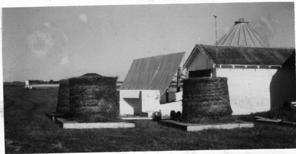
Figure 4. Large cylindrical bales drying facility: Drying Test No. 1, August, 1977.
