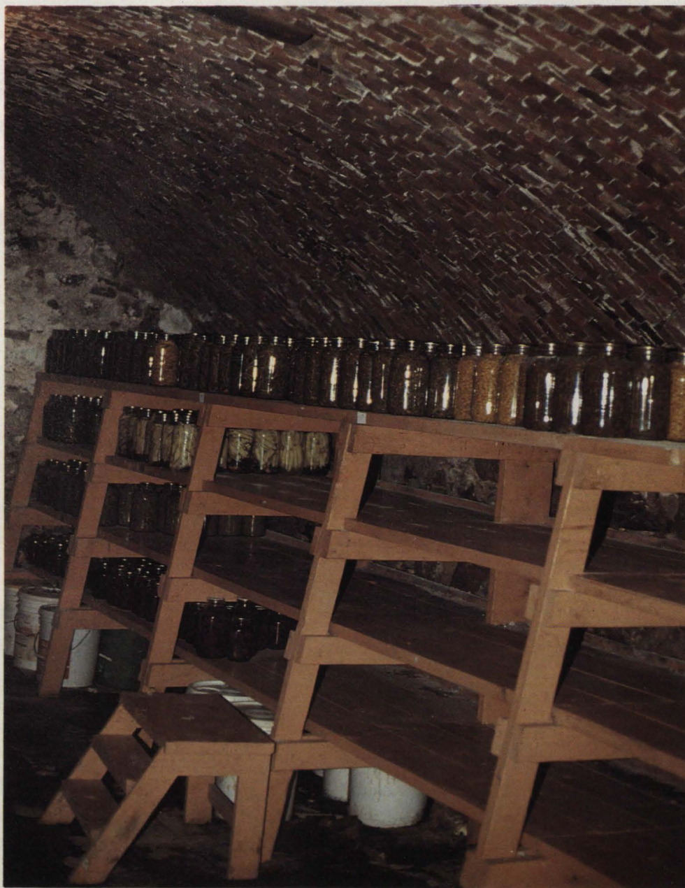
Bon Homme Colony, the oldest Hutterite colony in the United States, was founded in 1874. Today, many of the old structures are still useful. This storage cellar in one of the colony's older buildings features an arched brick ceiling.
