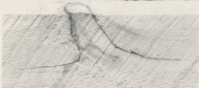
The defect produced in boards by branches. This is a loose knot.
