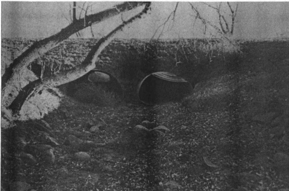
Plate H: Culverts from Outlet.
