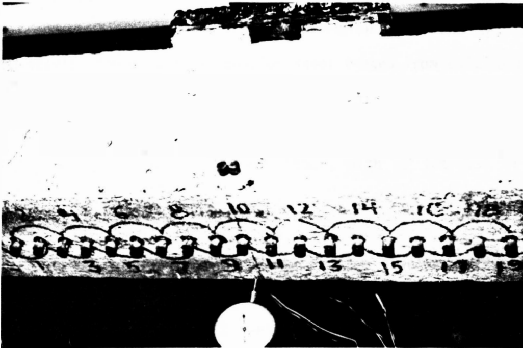
Figure 7.25. Cracks in fibrous concrete.
