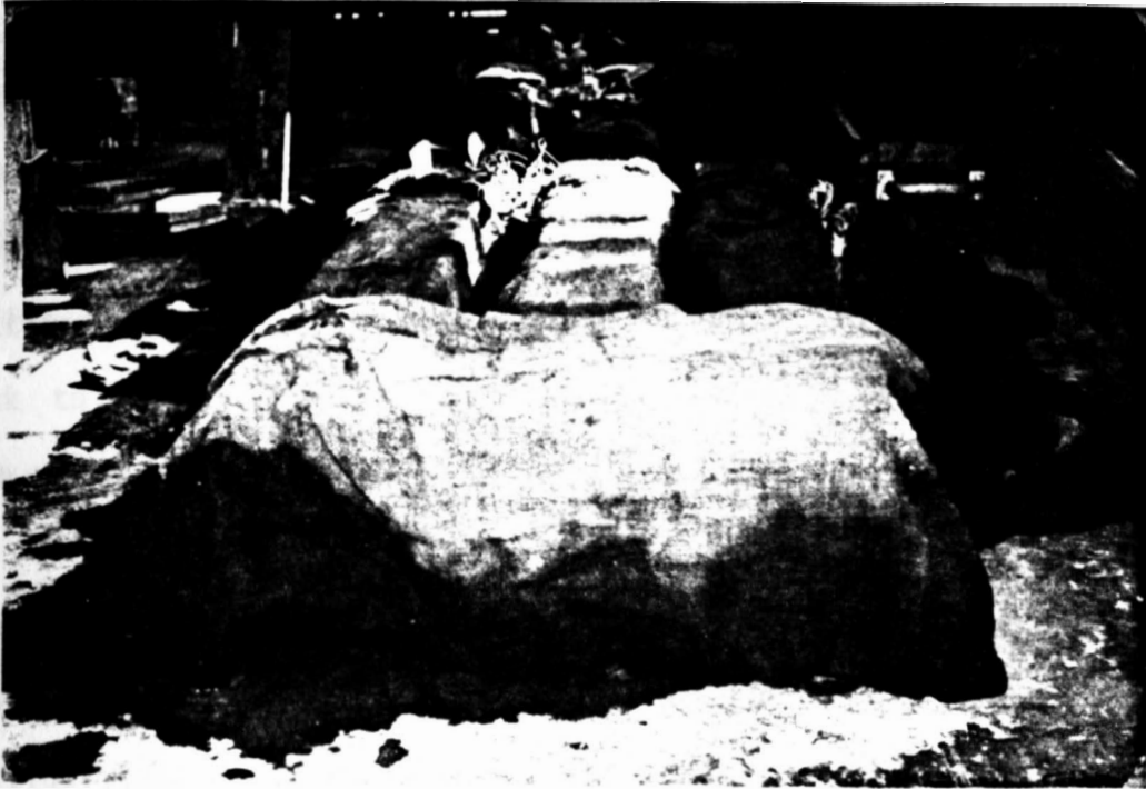
Figure 3.11. Concrete curing.
