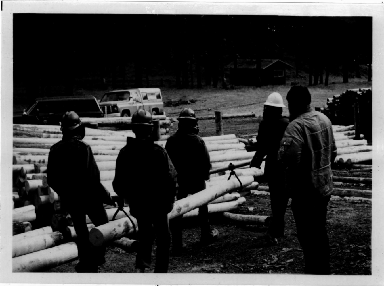
Figure 12 - New Building Construction Phase at Custer State Park (Photo Credit: Custer State Park)
