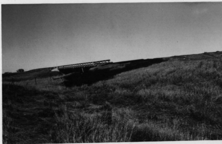
Fig. 13. Grass Fire Area.
