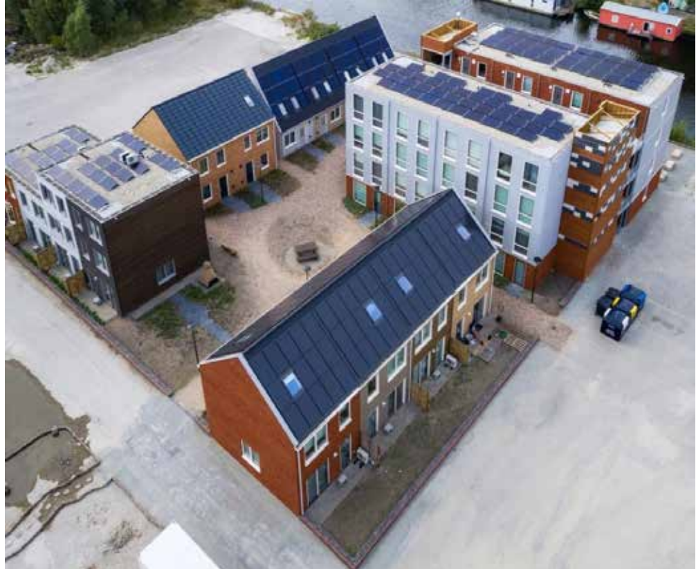
Figure 4.1 Loskade project in August 2019
