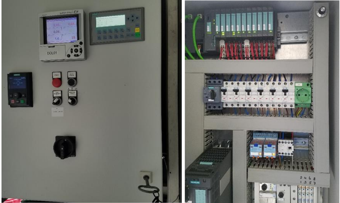
Figure 3-2 Dial for the Flow of Feedwater through the Membrane
