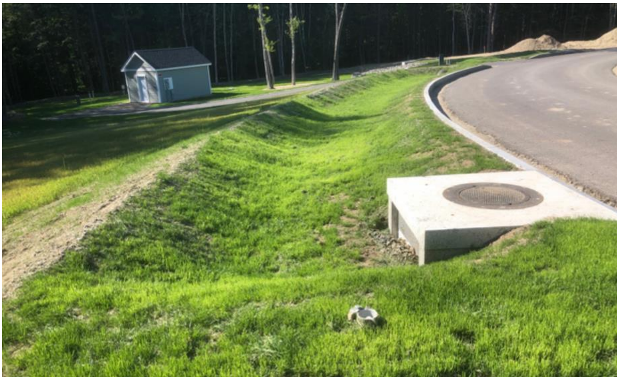
Figure 4.8 – Residential Bioswale with Pretreatment
