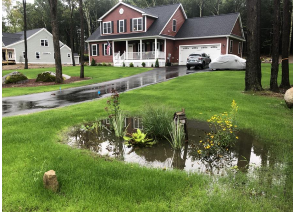
Figure 4.5 – Residential Raingarden for Rooftop and Driveway Runoff
