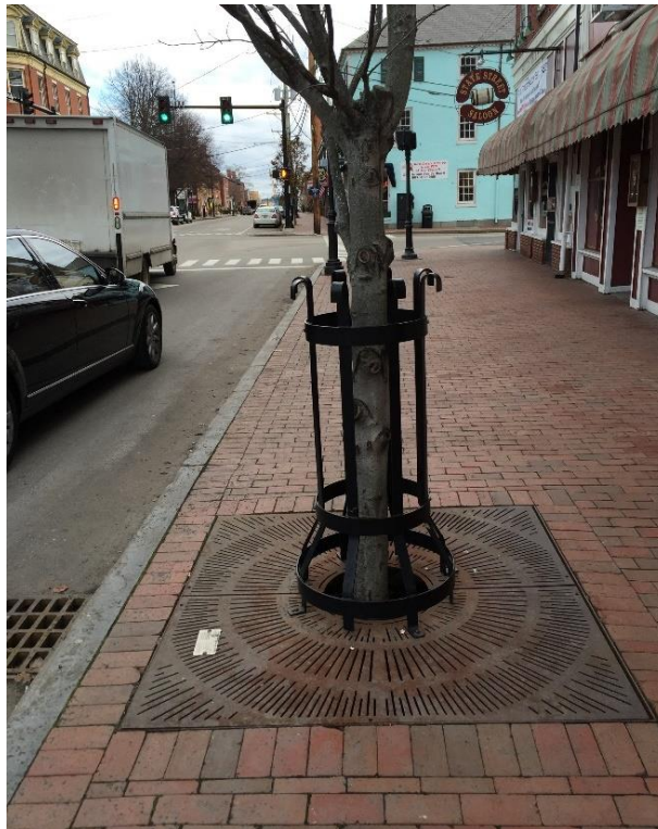
Figure 4.6 - Stormwater Tree Planter Combined with Catch Basin
