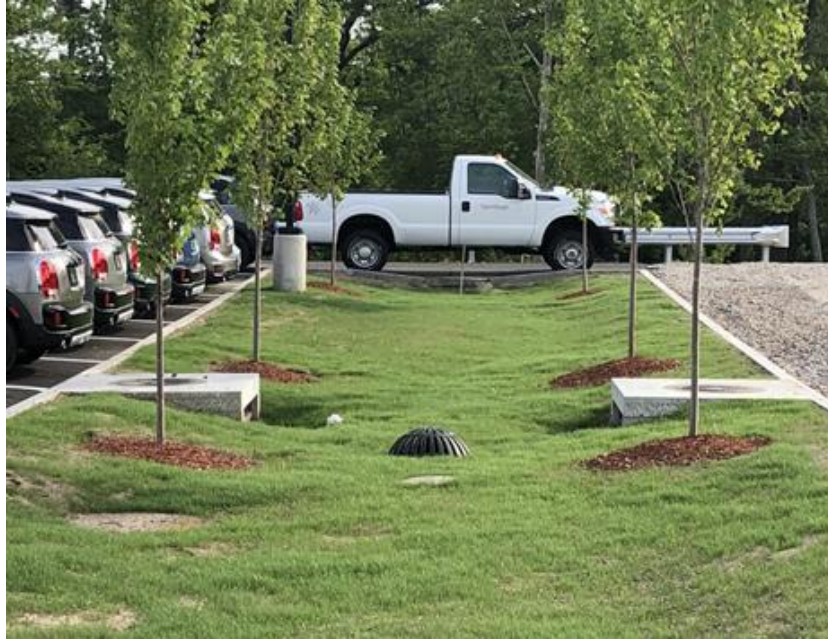
Figure 4.7 – Commercial Parking Lot Bioretention with Pretreatment
