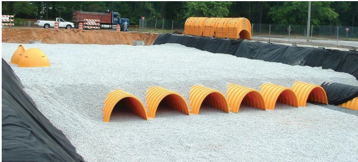
Figure 4.11: Subsurface Infiltration with Chambers and Pretreatment
