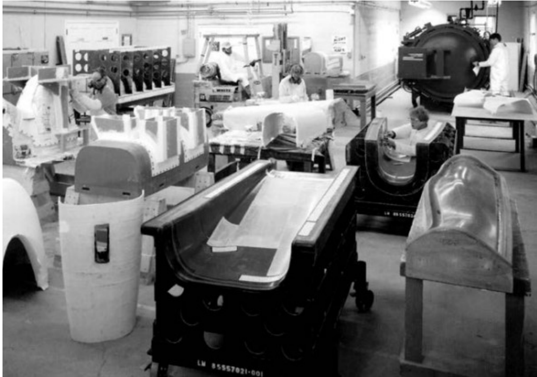
Figure 2.5 Master models and laminated molds (taken from [5])
