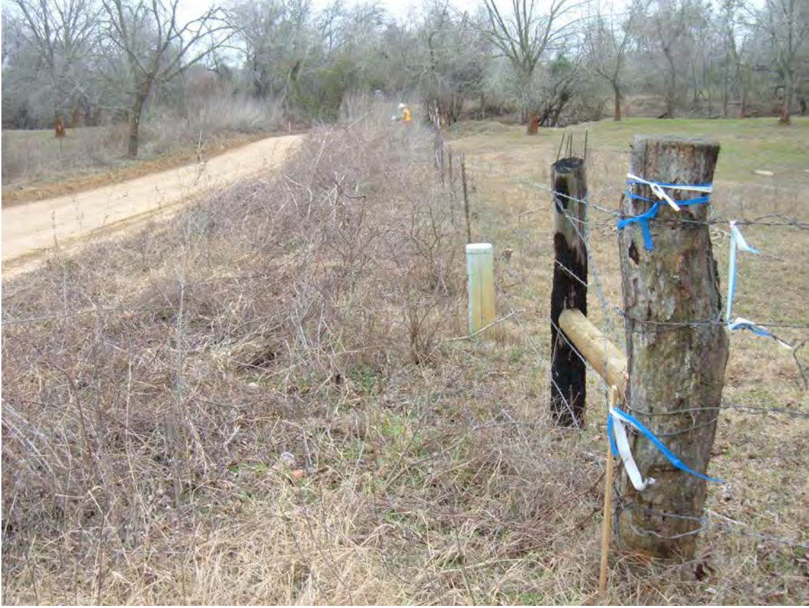
Figure 11. Overview of buried utility along fence line along western approach; facing east.
