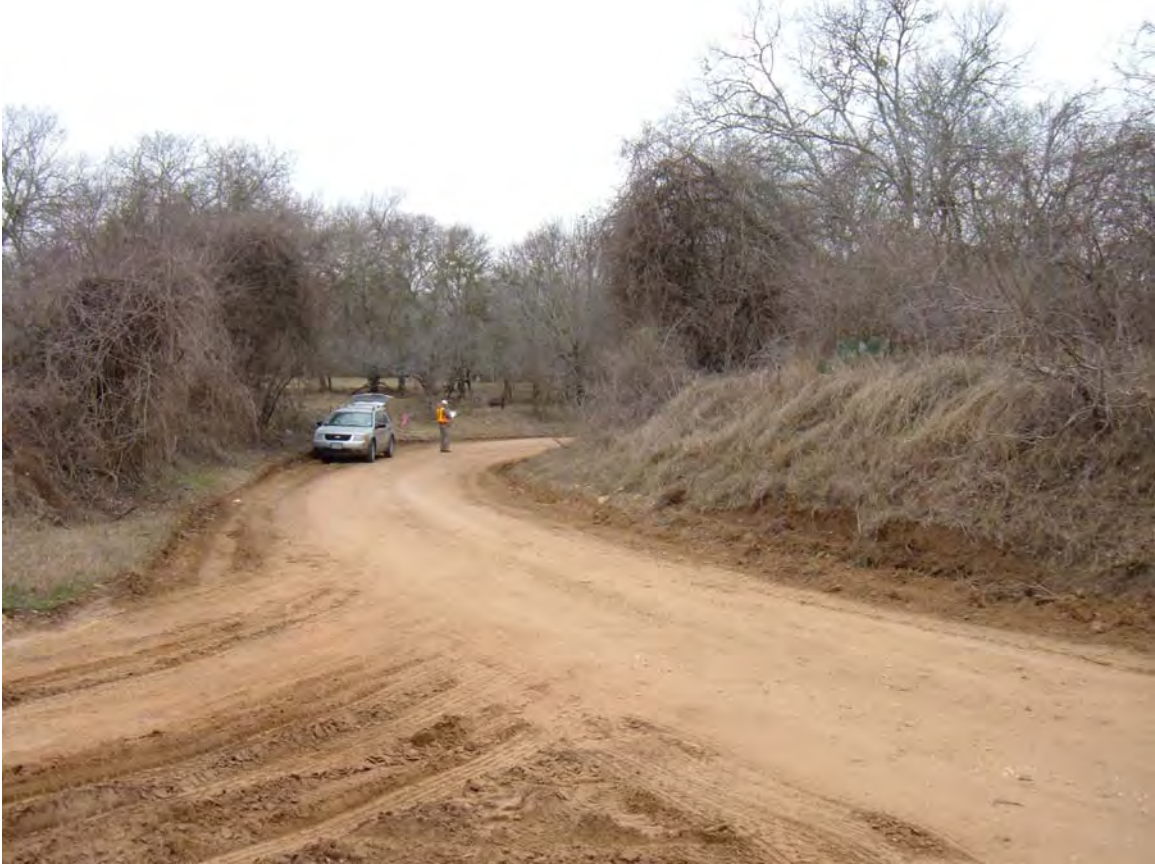
Figure 9. Overview of road cut below grade along eastern approach of project area; facing south.
