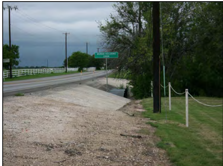
Figure 6. Overview of concrete and gravel apron along east side of roadway; facing north.
