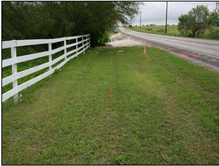
Figure 7. Note orange buried utility paint markings along fence line; facing south.
