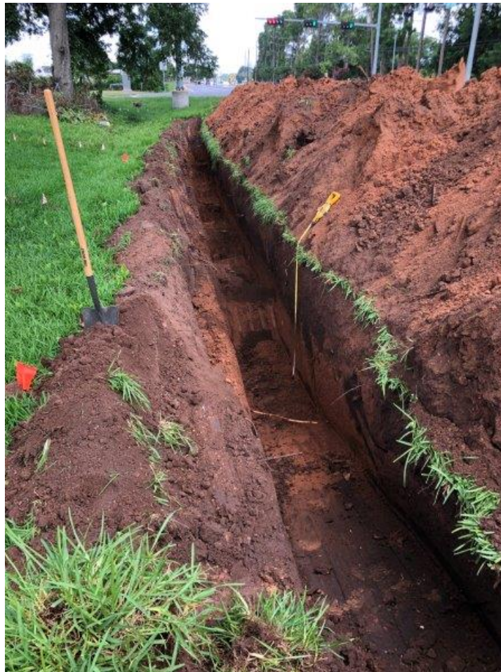
Figure 8. View of excavated trench, facing east.
