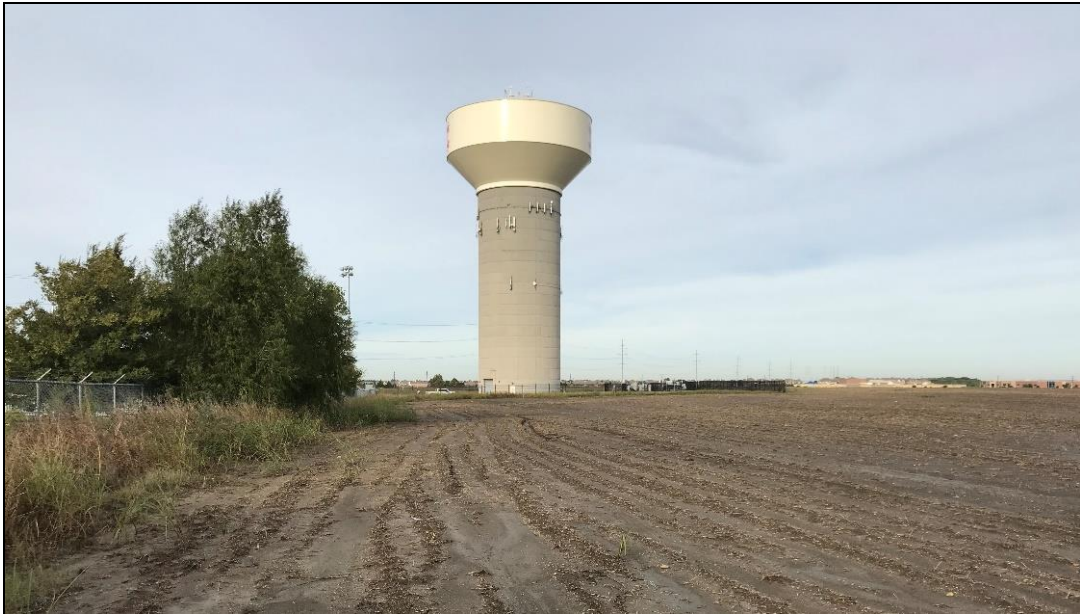
Figure 10. Overview of APE with water tower, facing west
