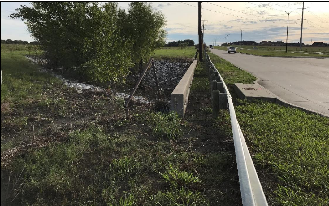
Figure 7. Overview of APE with concrete culvert, facing east
