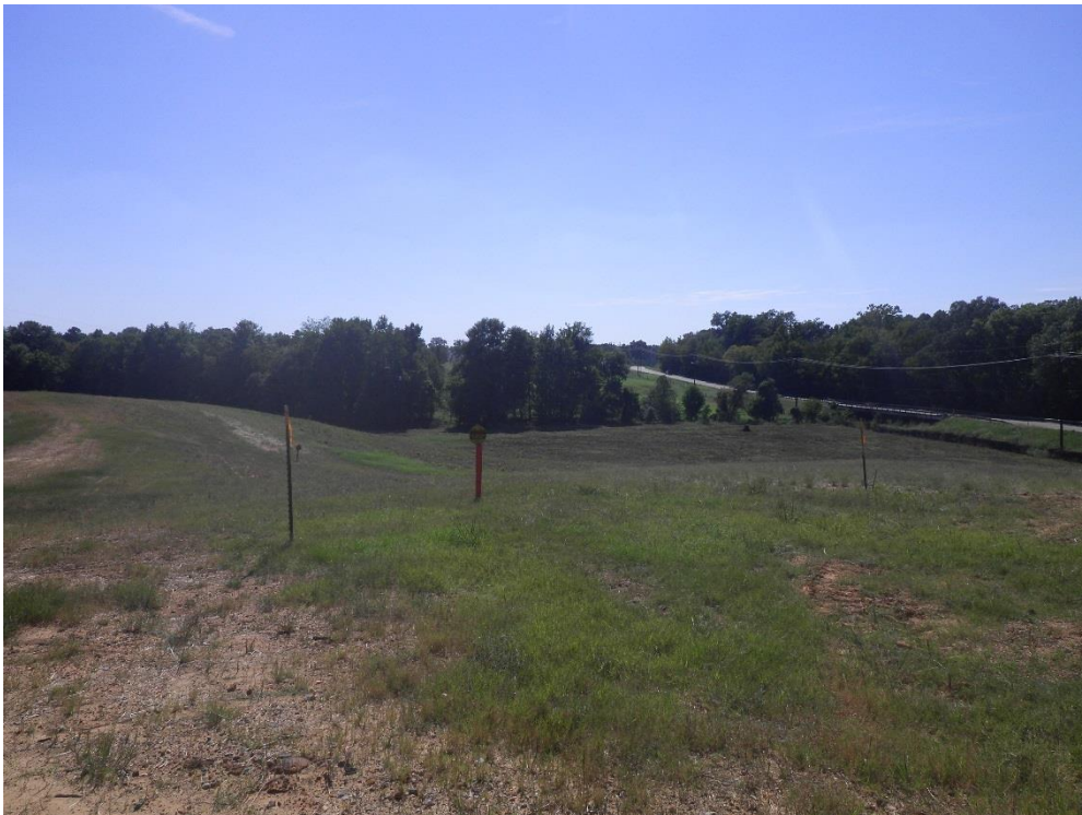
Figure 19. View toward Exxon pipelines; alignment identified by above-ground caution markers; view to the southwest.
