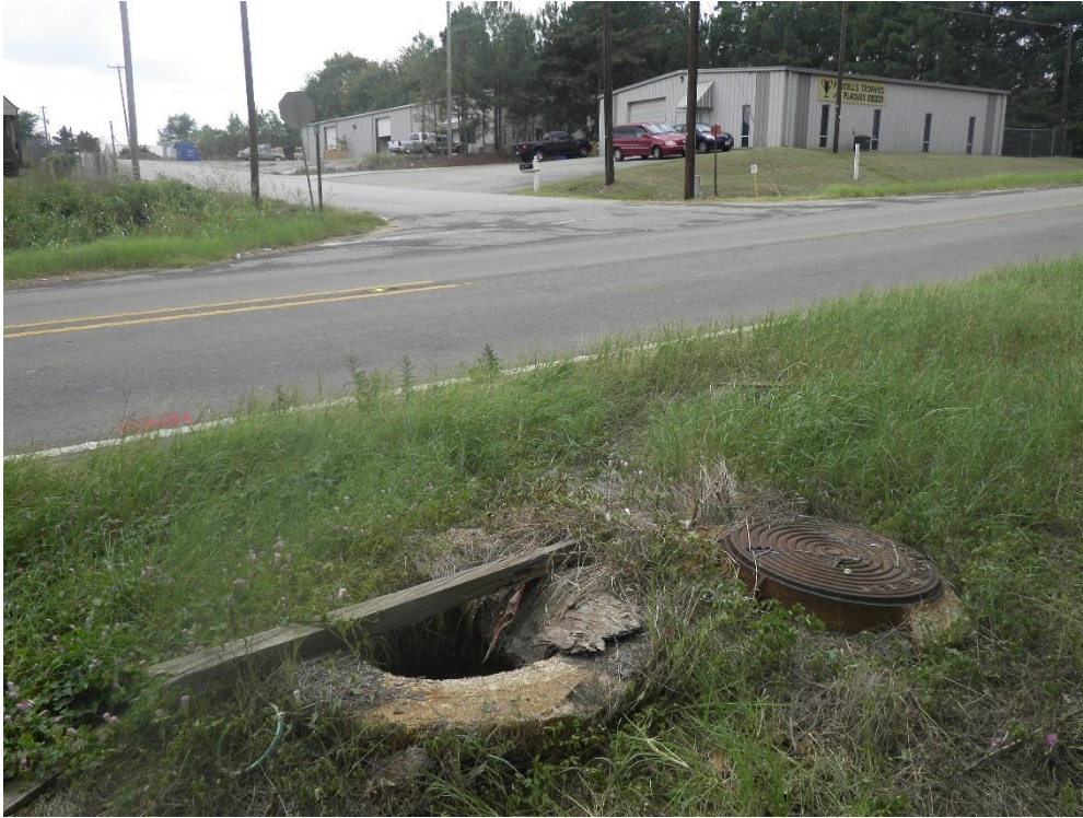
Figure 5. Evidence of subsurface utilities near unnamed drainage in APE with typical commercial enterprises in the background; view is to the north.
