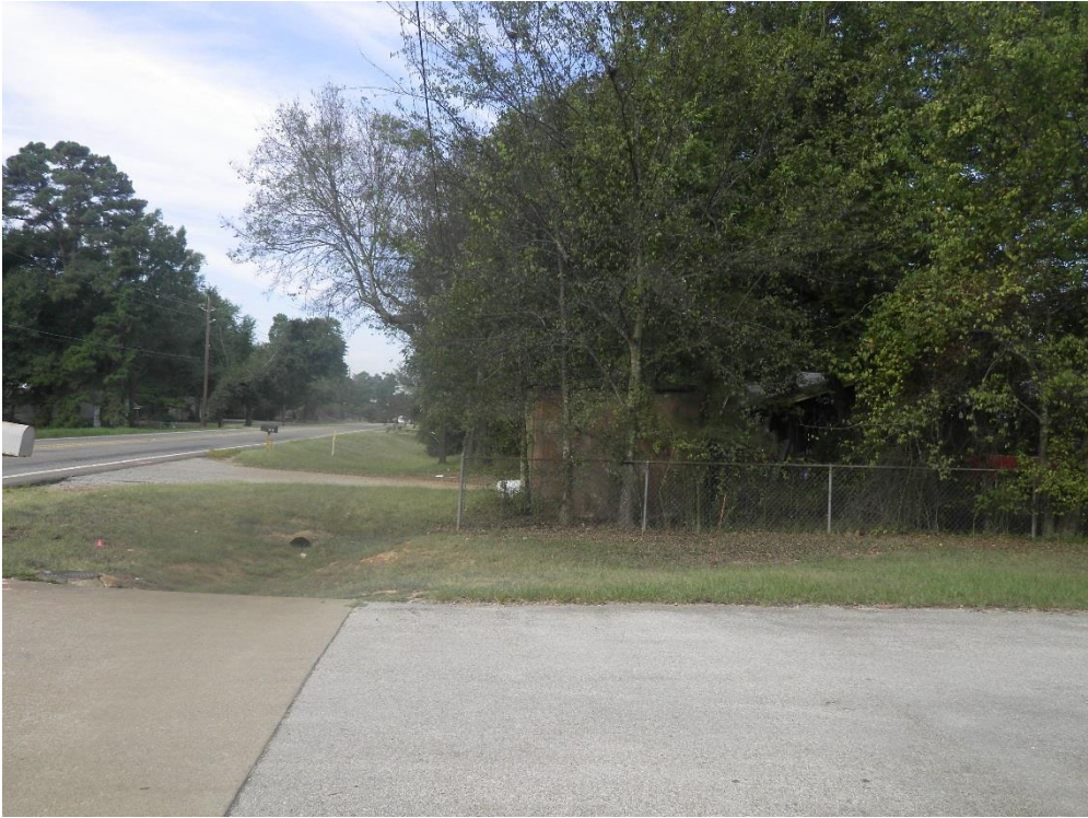
Figure 7. Area where the roadbed has been built-up; view is to the west.
