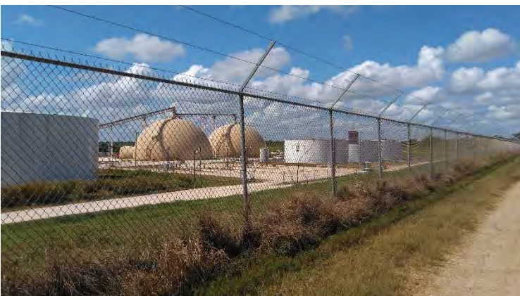
Photograph 5 - Eastern portion of the APE, view to the southwest.
