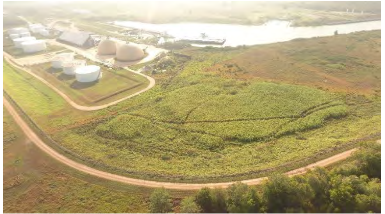
Photograph 2 – Central and eastern portion of APE, view to the east.
