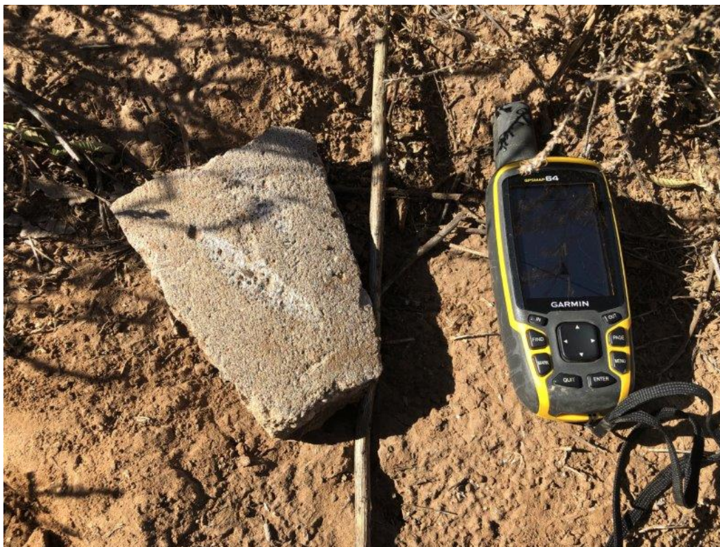
Figure 10. Concrete fragment observed adjacent to APE
