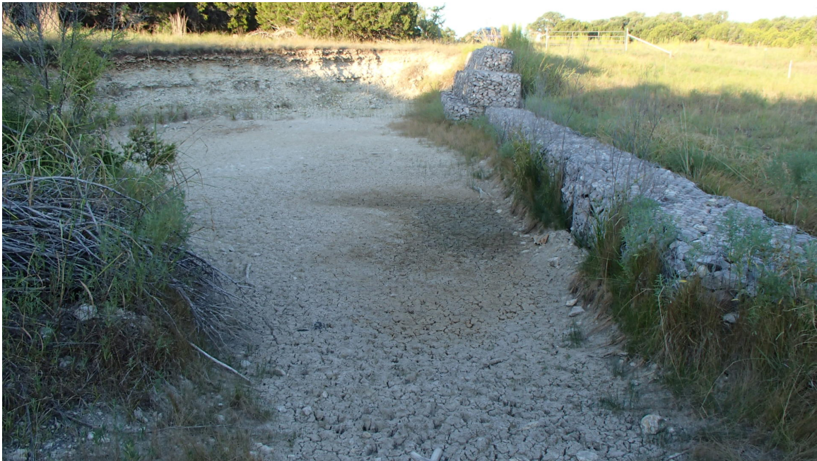
Figure 9. Man-made erosion control feature, facing northeast.
