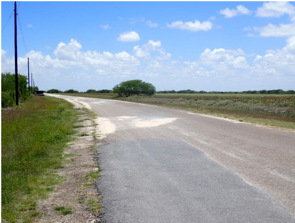
Figure 4-23. HR-01, Buena Vista Road, facing south from South Boundary Road
