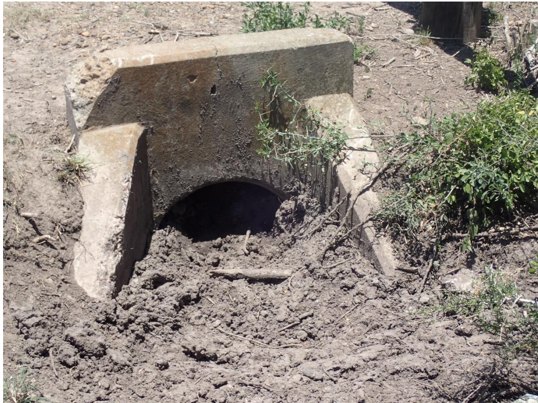
Figure 4-26. HR-04, culvert, south side of culvert, facing north
