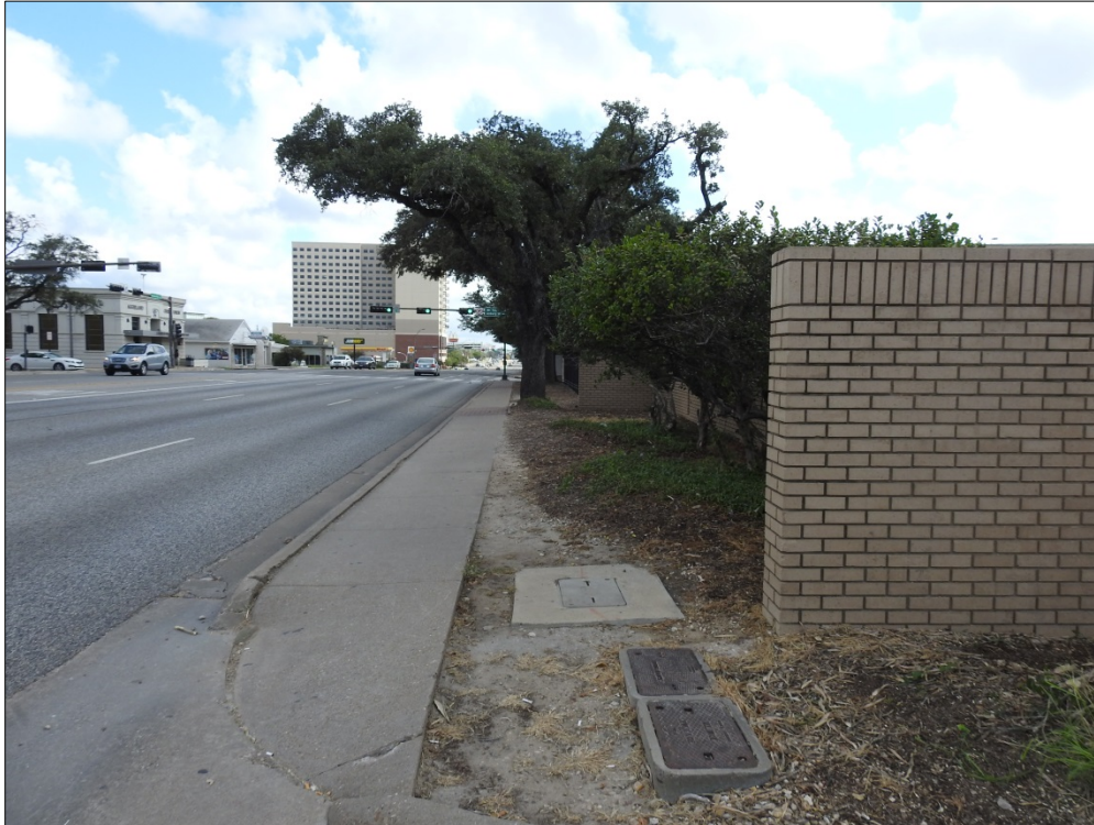
Figure 4-4. Photograph along South Side of University Drive Showing Buried Utilities in a Landscaped Area, Facing Northeast.
