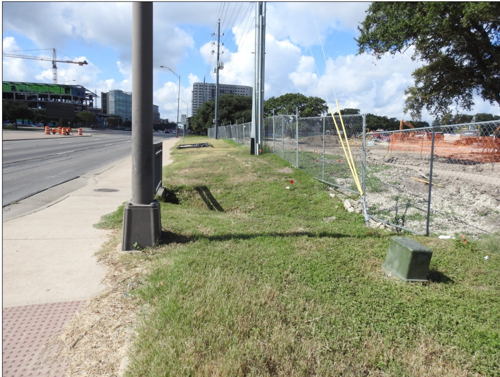
Figure 4-12. Numerous Utilities and Disturbance on North Side of University Drive, Facing Southwest.
