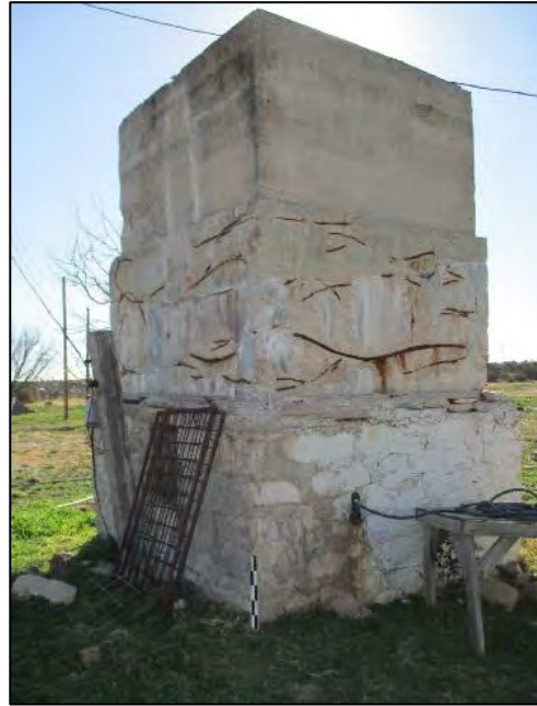
Figure 19. Feature 6 at 41UT147, facing southeast.
