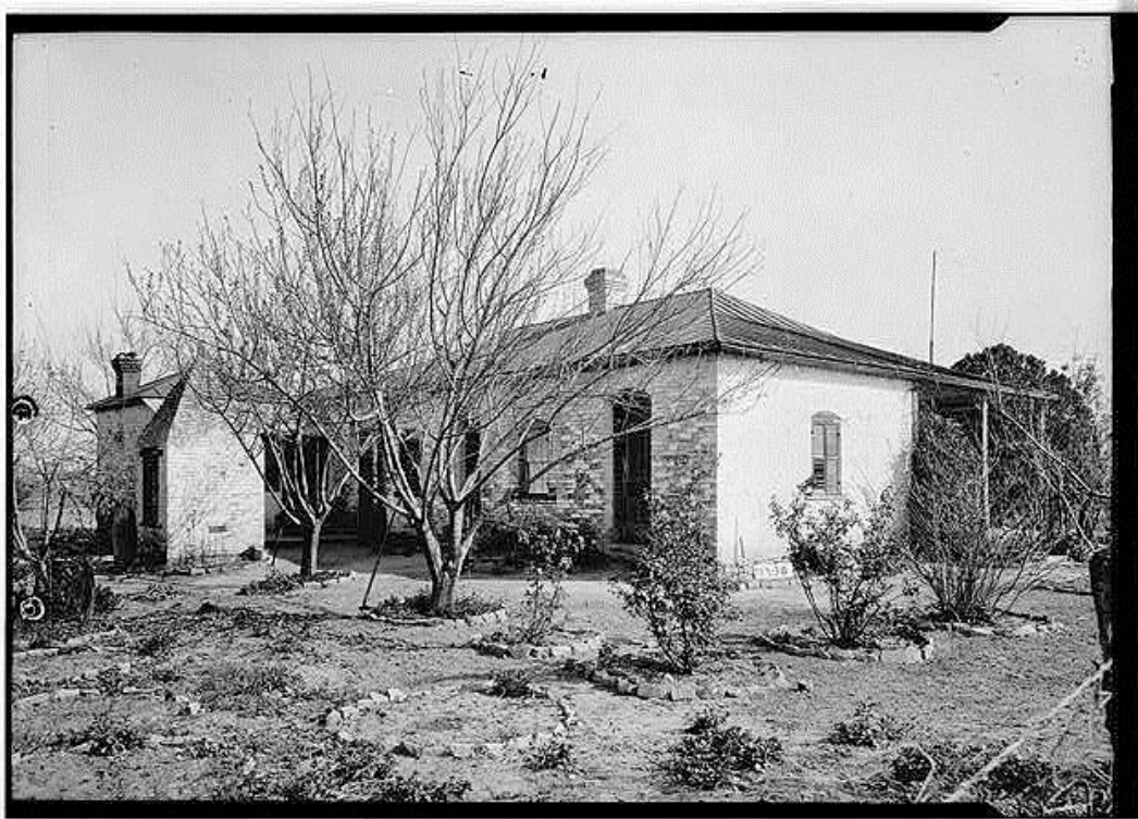
Figure 14. Northwest elevation (West side and North rear), Francisco Flores Ranch House, Floresville, Wilson County, Texas. Source: HABS/HAER/HALS Collection from the Library of Congress, photo by Arthur W. Stewart.
