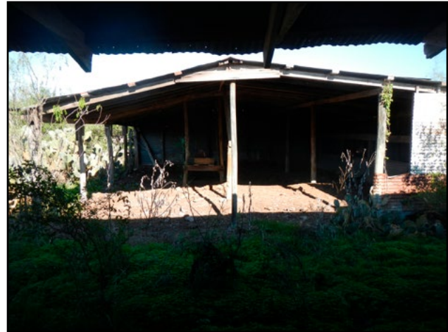
Figure 6.113. Feature HR02 on 41GU181, facing northwest.
