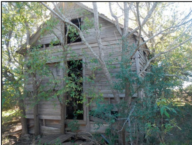
Figure 6.103. Feature HR02 on 41GU180, facing south.
