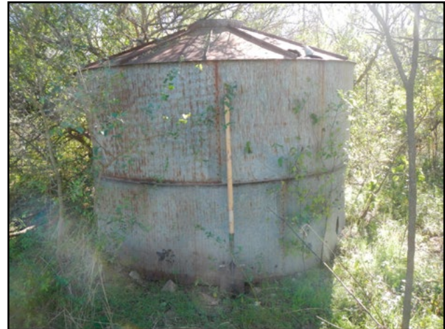
Figure 6.105. Feature HR03 on 41GU180, facing northwest.
