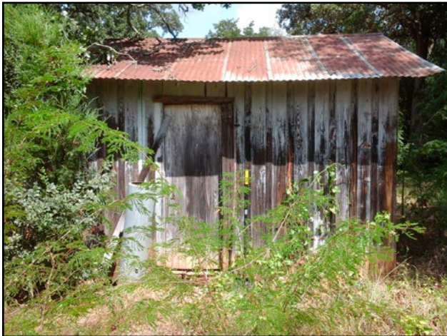
Figure 6.3. Overview of buildings on 41BU115, northeast elevation facing southwest.
