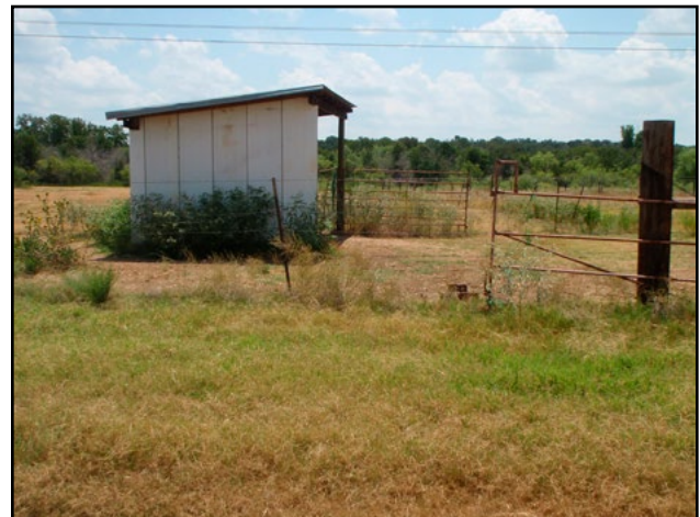
Figure 6.41. Existing shed within the boundaries of site 41BP920, facing west.
