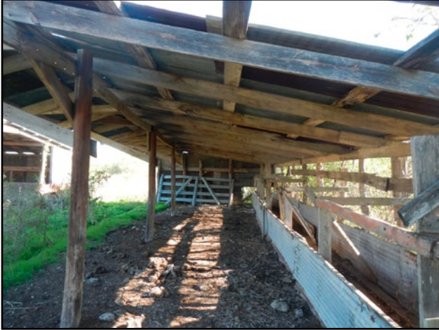
Figure 6.112. Feature HR01 on 41GU181, facing east.
