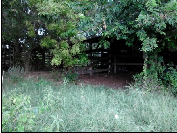
Figure 6.52. Extension of structure serving as livestock shelter and storage on 41CW162.
