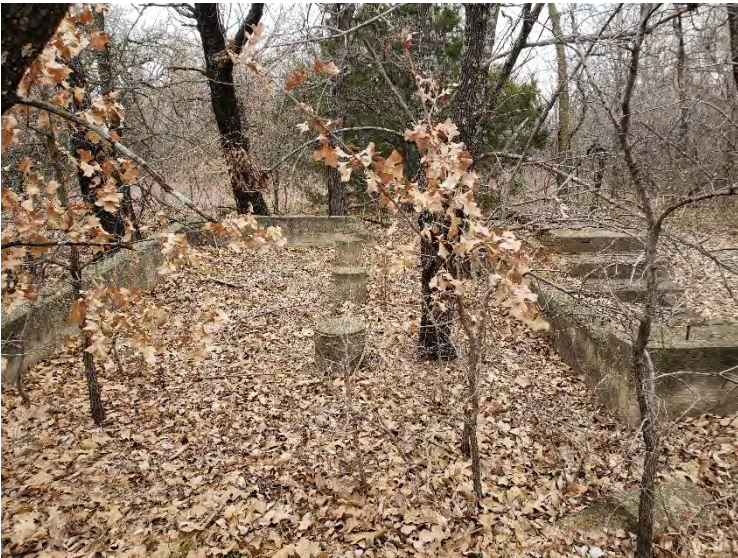
Photograph 51 – Site 41TR87: Feature D concrete footers, view to the north.
