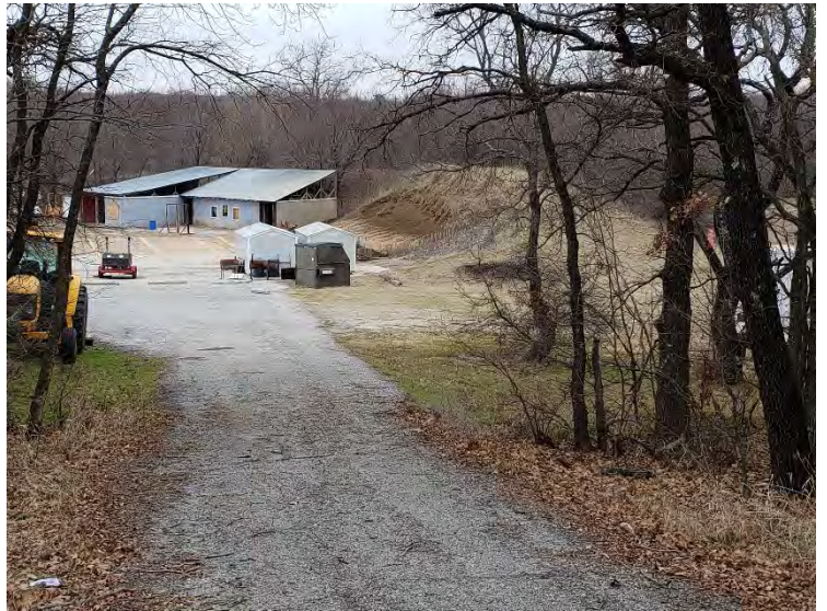
Photograph 28 – Gun range facility, view to the west.
