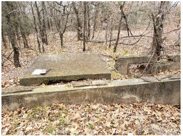
Photograph 50 – Site 41TR87: Feature D concrete footers, view to the west.
