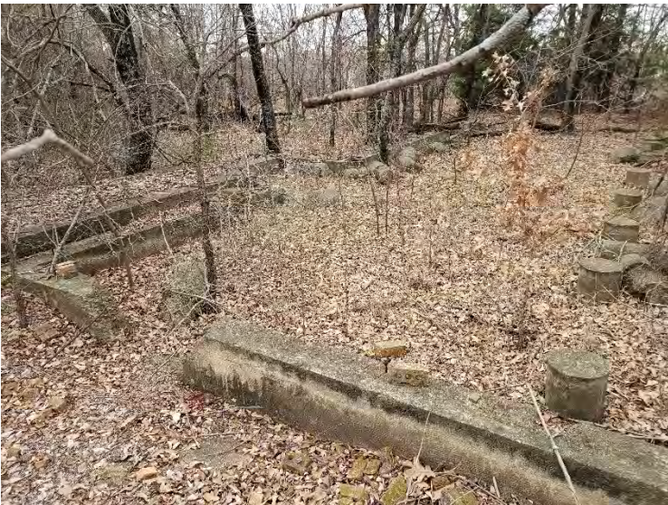
Photograph 53 – Site 41TR87: Feature D concrete footers, view to the southeast.
