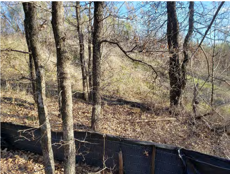
Photograph 47 – Fill from pad site, view to the south.
