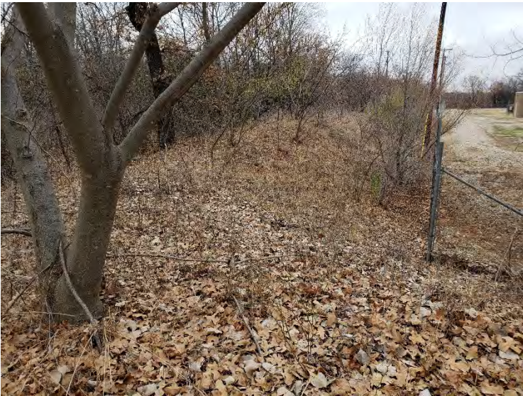
Photograph 45 – Earthen berm around pad site, view to the east.
