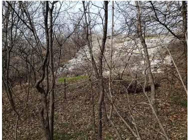
Photograph 46 – Rock rip-rap, view to the west.
