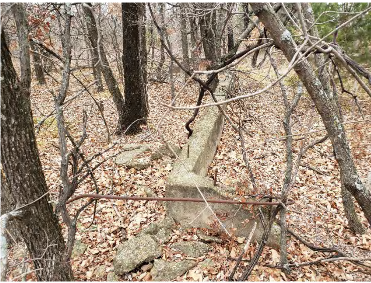
Photograph 49 – Site 41TR87: Feature D concrete footers, view to the north.
