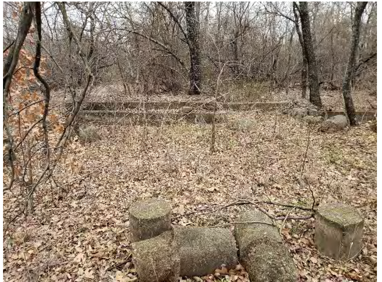
Photograph 52 – Site 41TR87: Feature D concrete footers, view to the east.
