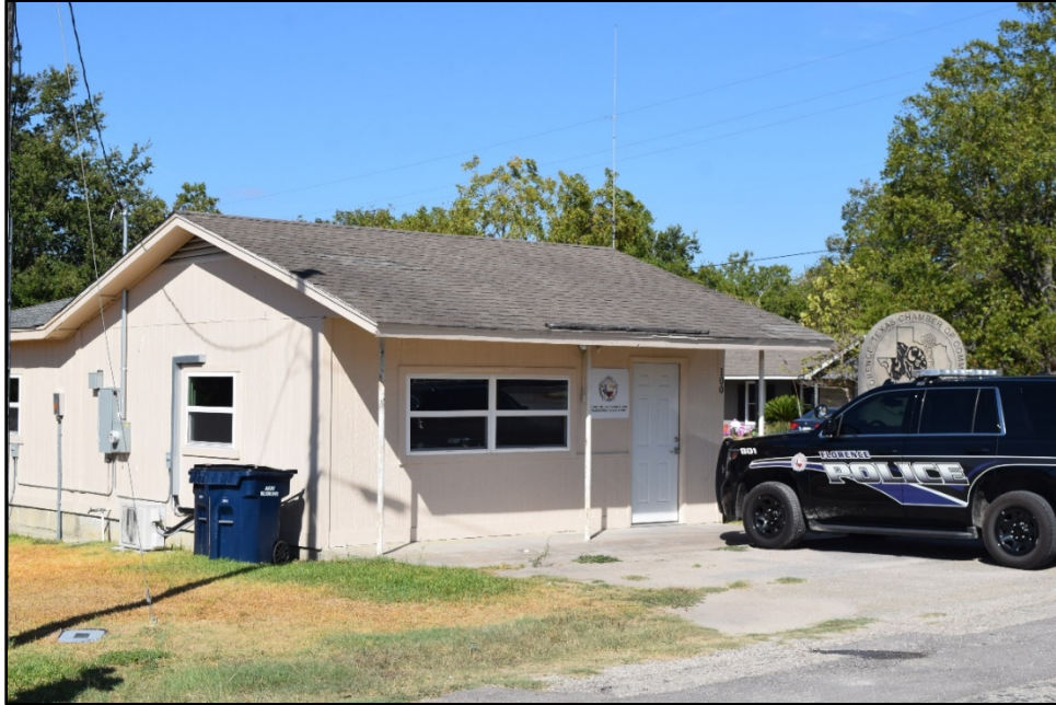
Figure 16. Chamber of Commerce, oblique, east (front) and south elevations, facing northwest.
