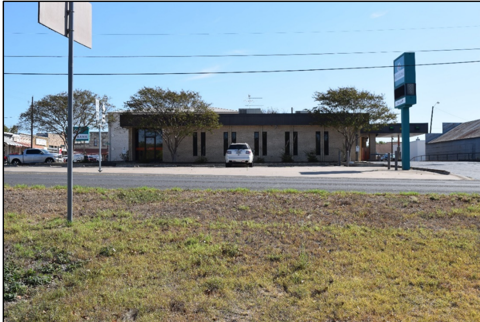
Figure 20. Modern bank building, corner of Main and Patterson, east of project area, west elevation, facing east.
