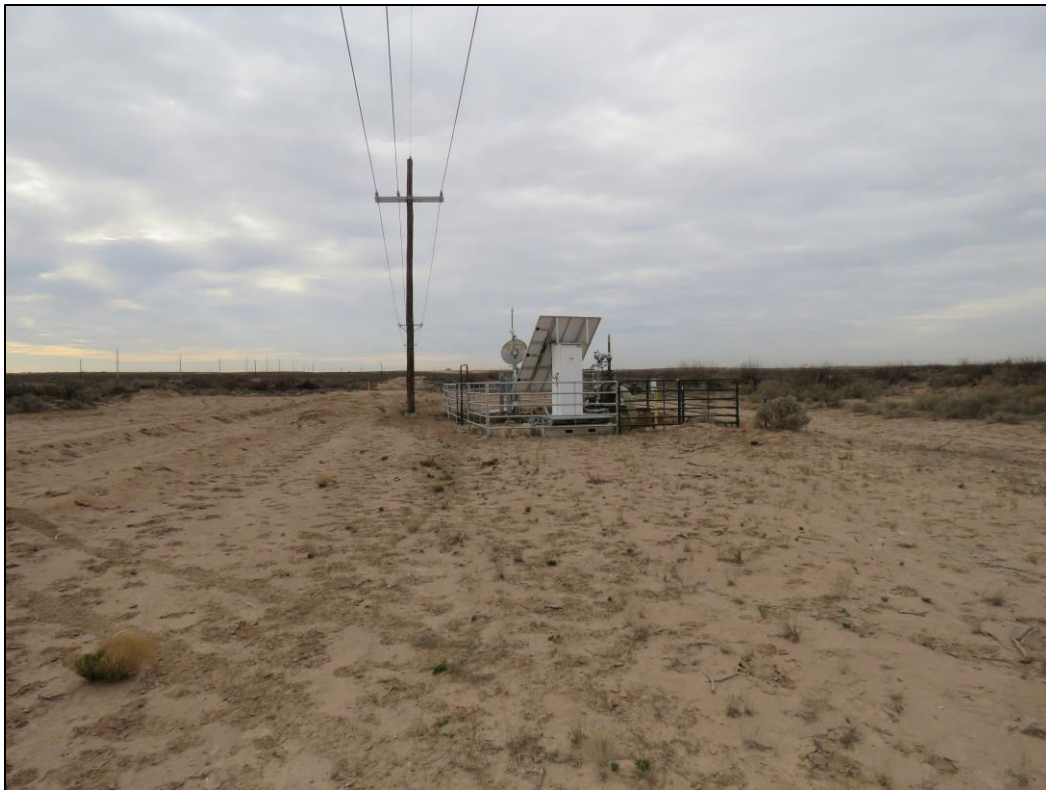
Figure 9: Example of pipeline corridor and telephone utility crossing the Route, looking south.
