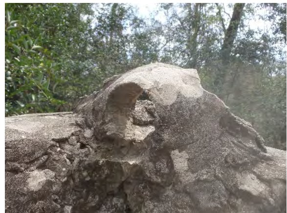
Figure 7-18. Detail of mortar roof bracket on Historic Age Structure 1.
