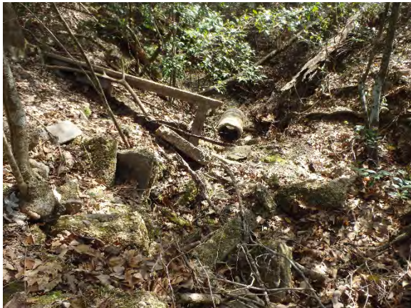
Figure 7-19. Typical example of concrete rubble deposited in erosional gully. View is to the east.
