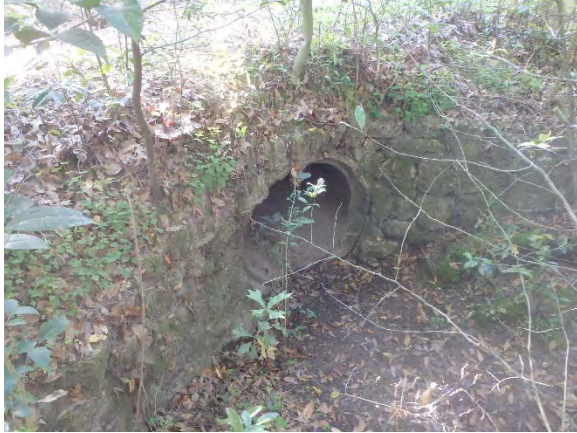
Figure 8-2. Historic Age Structure 4. View is to the southeast.
