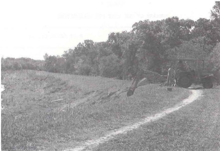
Figure 4b. Backhoe trenching at 41HR259.
