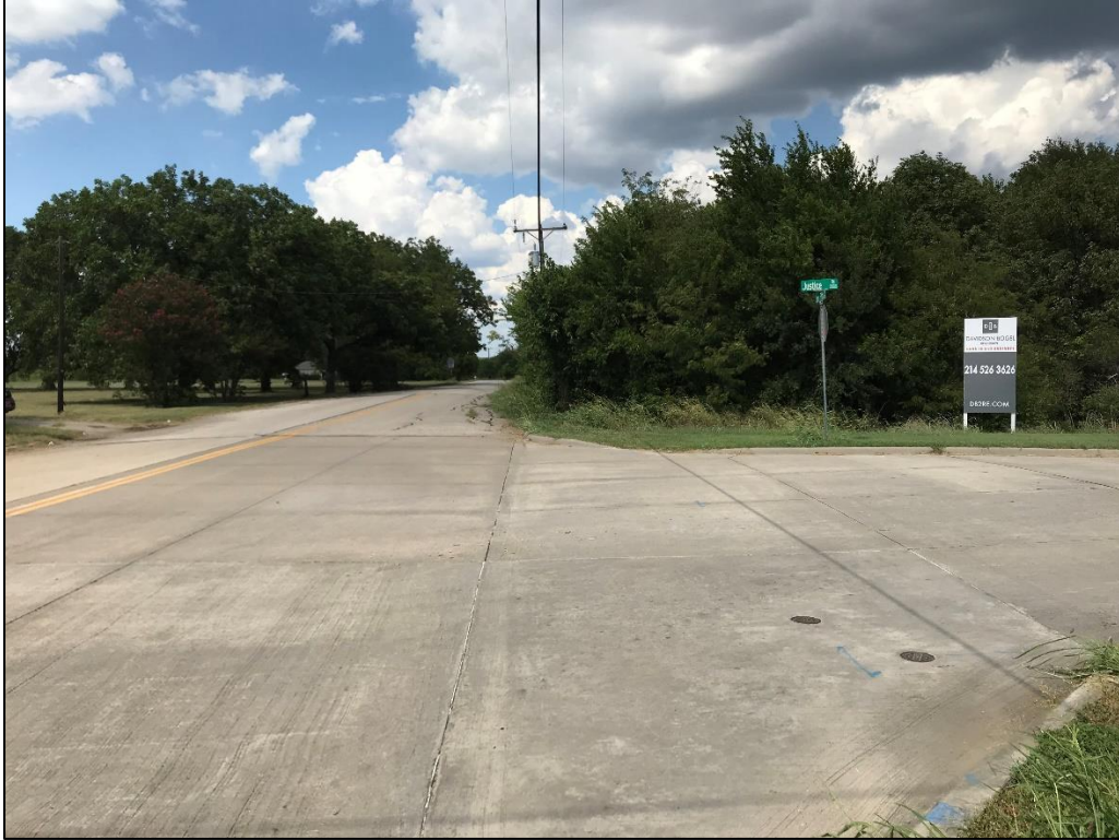
Figure 5. Transmission line easement at intersection of James Pitts Drive and Justice Road. Facing south.
