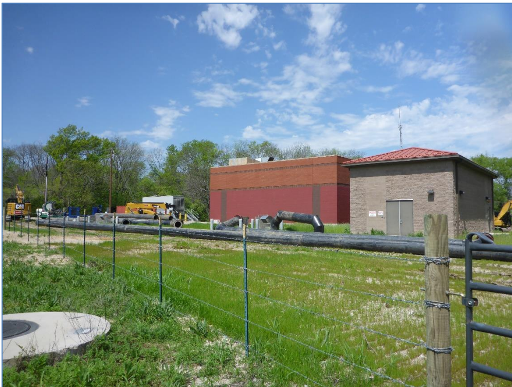
Figure 14. NTMWD maintenance facility construction disturbance in the northeast corner of APE; view northwest.
