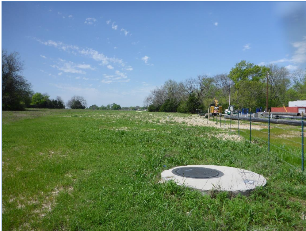
Figure 15. Sewer line disturbance at the northeast corner of APE; view west.
