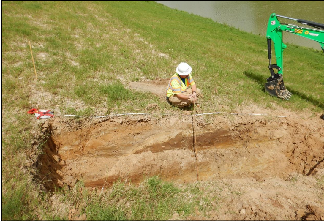
Figure 12. Trench 4 (facing west).
