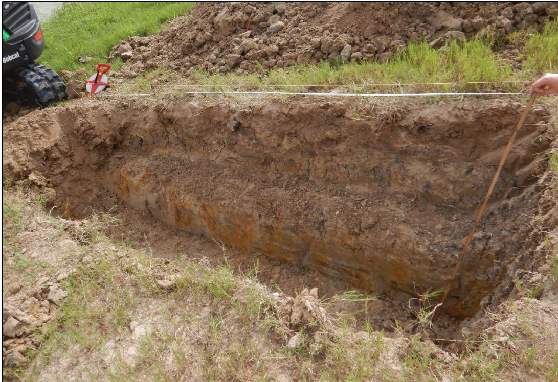
Figure 13. Trench 5 (facing east).
